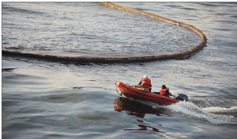
Members of Elastec/American Marine Inc. inspect a fire boom containing collected oil prior to conducting a controlled burn in the Gulf of Mexico on May 5, 2010. The U.S. Coast Guard, BP, and other federal agencies conducted controlled burns to aid in preventing the spread of oil following the April 20 explosion on the Mobile Offshore Drilling Unit Deepwater Horizon . Navy photo by Petty Officer 2nd Class Justin Stumberg
