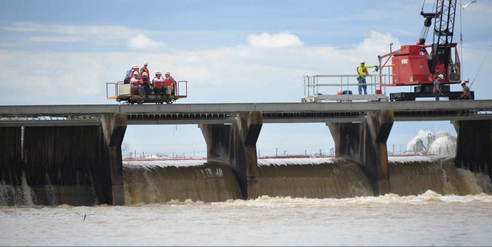
Located about 12 miles west of New Orleans, the Bonnet Carré Spillway is a flood control operation that allows waters from the Mississippi River to flow into Lake Pontchartrain. In 2019, for the first time in history, the spillway had to be operated twice in one year. U.S. Army Corps of Engineers photo
