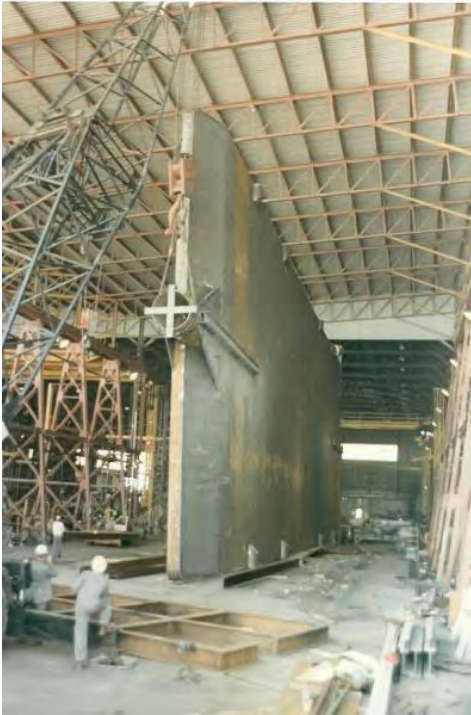
At left, large platform is being flipped inside Thompson Metal Fab's shop.
