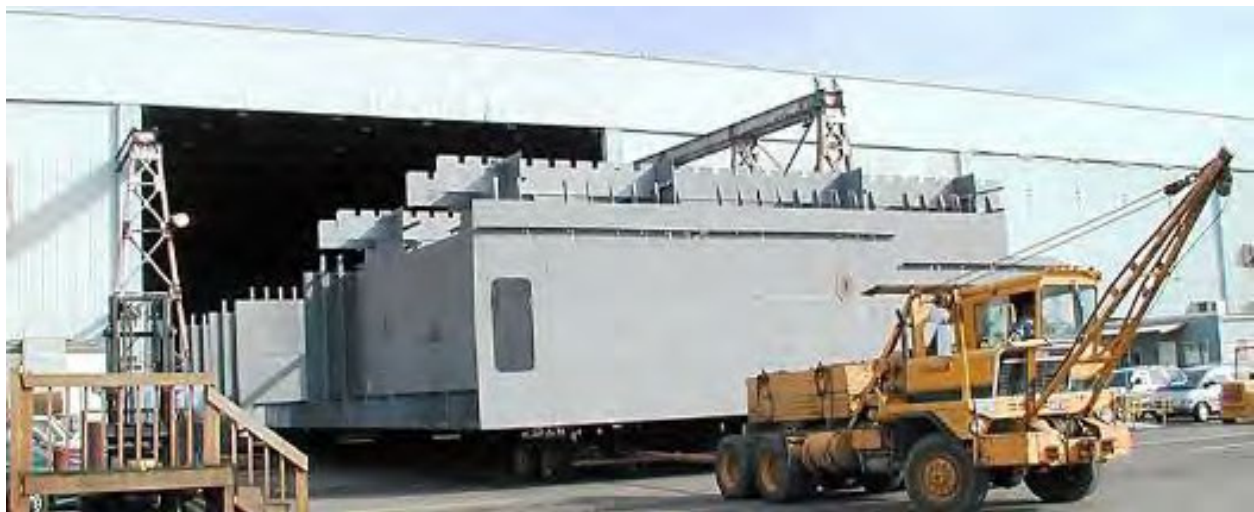
Shown above and below is a modular segment of the Power Barge fabricated by TMF. Segments were pre-fabricated in the shop before being assembled in Thompson's yard. The final assembly was 105' W x 30' H x 284' L
