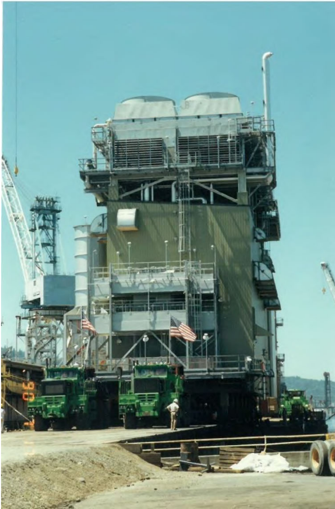
This massive process module is being loaded out for delivery to the North Slope of Alaska in July 1990. This industrial equipment rivals the size of most downtown buildings and is representative of the equipment currently being requested for North Slope expansion projects.
