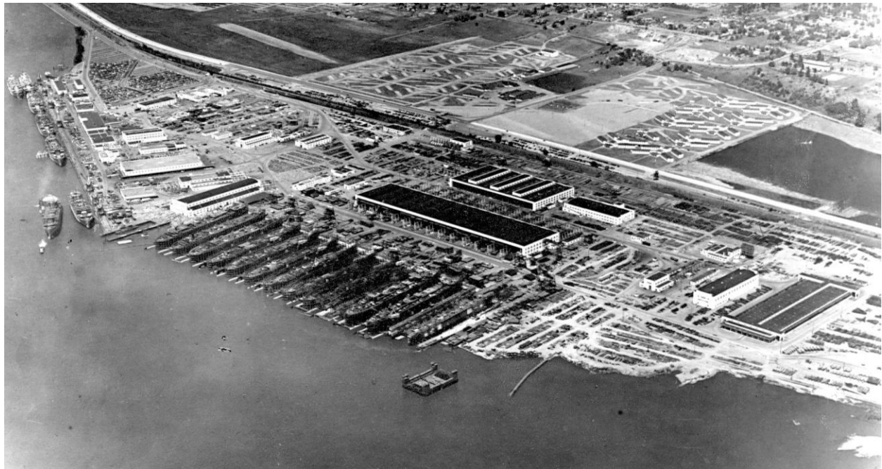
Building 40 and 41 of current day Thompson Metal Fab is shown prominently in the middle of this picture. At the time this picture was taken (circa early 1940's) the building and entire industrial area would have been known as Kaiser's Vancouver Shipyards.
