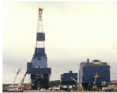
Rig 245 shown here at the assembly yard. When fully raised, the mast hangs high in the Vancouver, WA skyline.
