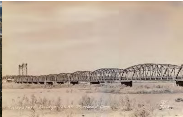
Original span of the Interstate Bridge opened 1917 – shown here in 1931.
