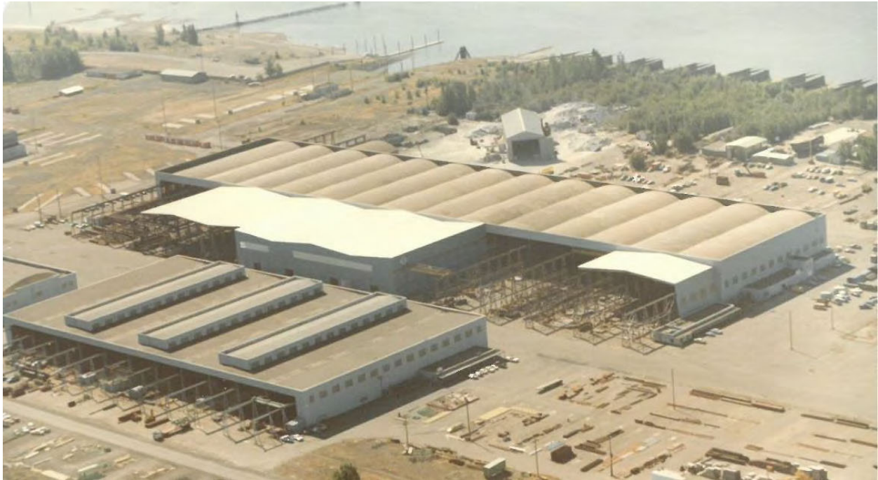
Taken in the early 1970's, the photo above shows Thompson Metal Fab shortly after closing the original facility in Portland and moving to Vancouver. Thompson added fiberglass roofing and walls to bays 5 through 9 to create an enclosed space. The land has been developed quite a bit in the last 40-years (including improvements to the roll-on/roll-off barge slip), but the building remains virtually the same.
