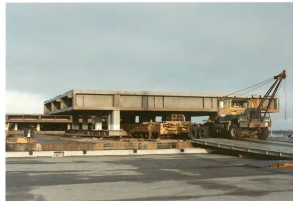
The platforms (seen left) were delivered by barge to Alaska where high capacity trucks and dollies (shown above) off loaded the structures for delivery to the jobsite.
