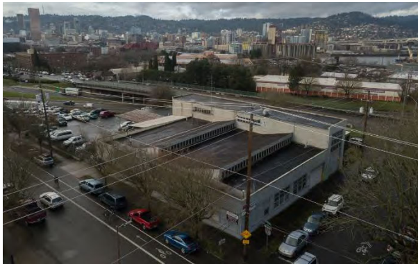
The original Thompson Metal Fab facility, shown in 2018. Thompson moved from this location and to Vancouver in the early 1970's. The old facility has since been demolished, making way for the brand new Meyer Memorial Trust building.
