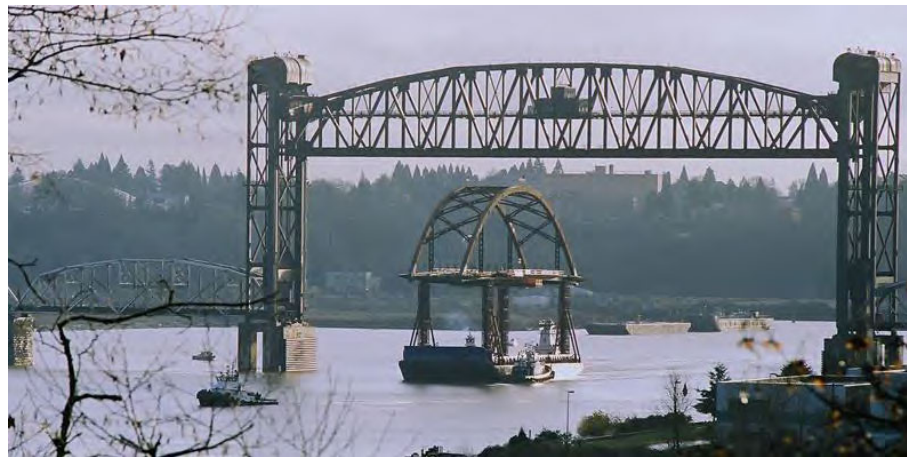
Image above shows the Sauvie Island Bridge being shipped to the jobsite via barge on the Willamette River and passing under the Burlington Northern RR Bridge in Portland, OR. Delivery of steel for the new Burnside Bridge would take a similar approach, due to the limited area for construction at the jobsite in downtown Portland, OR. Bridge steel coming from the Columbia Business Center would pass under the Interstate Bridge to reach the jobsite.
