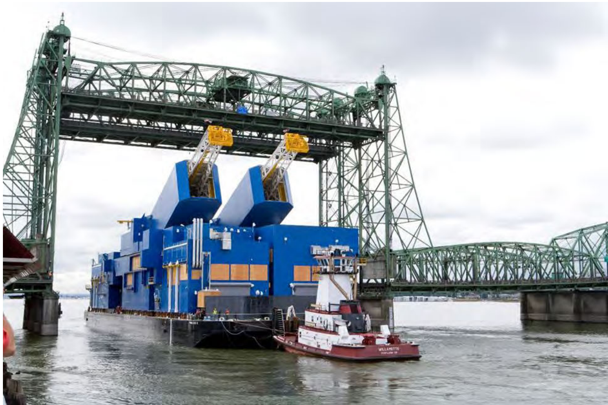
Picture of the Interstate Bridge in 2011 showing both the original Northbound span (background) and the second span (foreground) which opened in 1958 to traffic in both directions. In 1960, the second span was dedicated to Southbound traffic only. (Photo shows TMF manufactured drill rigs, AADU Rig 272 & 273 for Parker Drilling)
