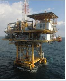
OCS facility, more commonly referred to as a fixed platform, consists of a bottom bearing rigid structure extending to the seafloor. Often the portion of a fixed OCS facility visible above the surface of the water is a small fraction of the overall structure. A topside "platform" is installed on top of the structure (**image above**).
