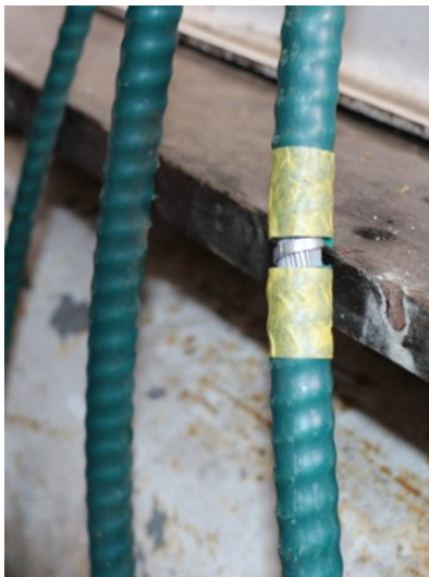
Figure 20: Section of conduit cover removed. Credit: CG.
