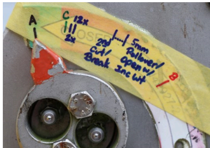
Figure 39: Locking shaft positions observed: 2 nd Cut/Break - position upon break of the polyethylene & separation of cable conduit "B" - open position with no load Rollover - locking shaft forced to open with increasing weight Dots: positions that hook supported the test weights applied; locking shaft is shown in the closed position (picture taken after testing). Credit: CG.
