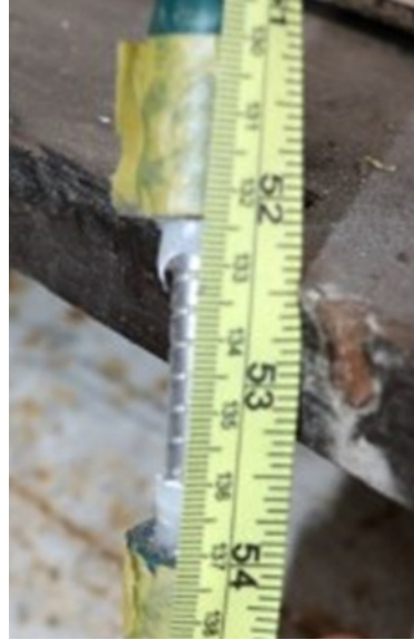
Figure 32: Conduit separation upon polyethylene liner breakage (closing action). Credit: CG.
