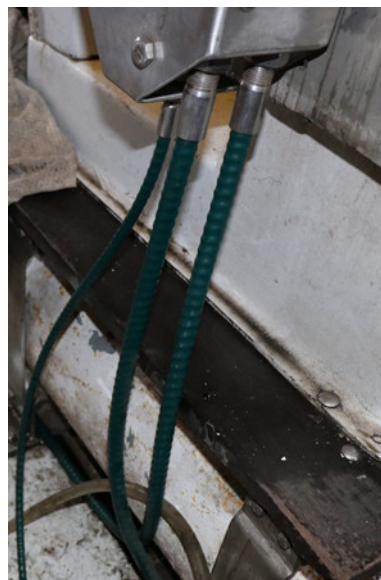
Figure 9: MSTC Lifeboat 1 cable routing at release unit. Credit: CG.
