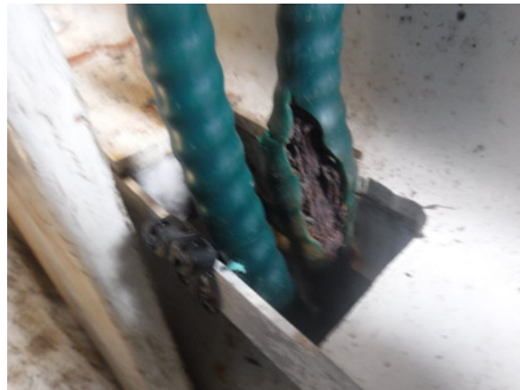
Figure 19: Condition of the aft hook control cable & location in relation to the bottom of the coxswain's console as documented Jun2019, prior to the incident. Credit: Palfinger.
