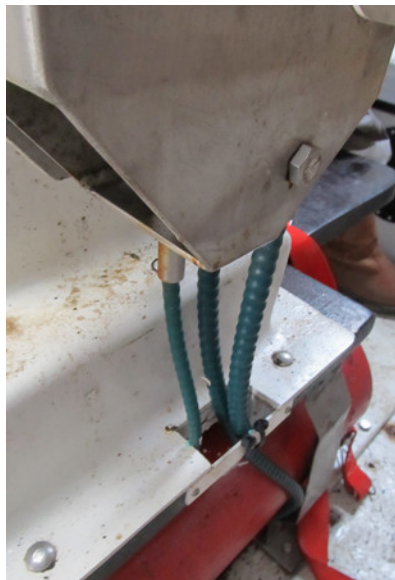
Figure 8: AUGER Lifeboat 6 cable routing at release unit (circa 2014). Credit: Shell.
