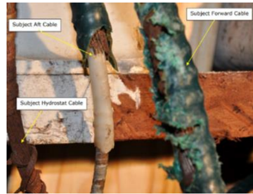
Image 7: Photograph of aft control cable after casualty. Photograph documents separation of three layers of the conduit: the green plastic cover; a steel wire; and a white polyethylene liner. Credit: DNV-GL.
