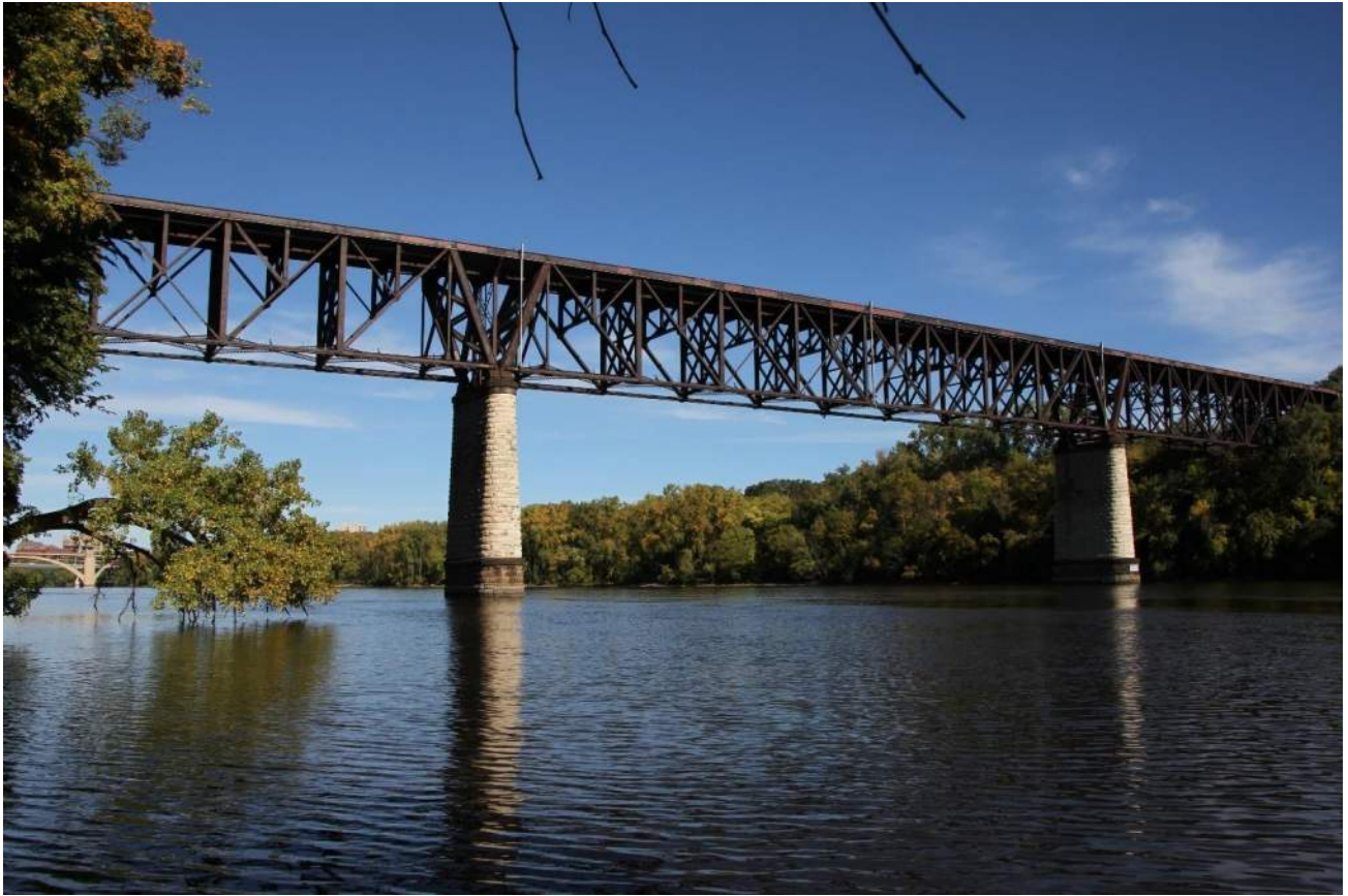
Exhibit B1: South Elevation of Truss Spans
