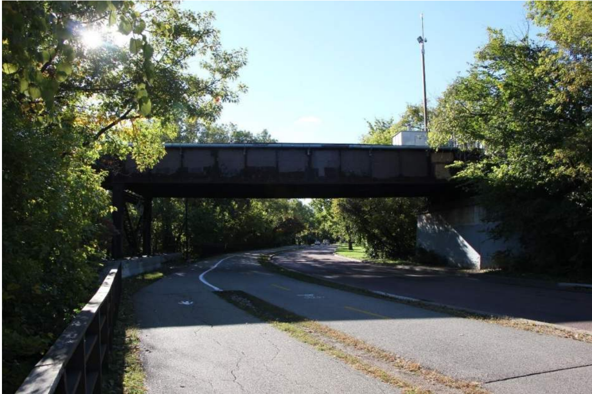
Figure 4: West Approach, Span 1 looking south
