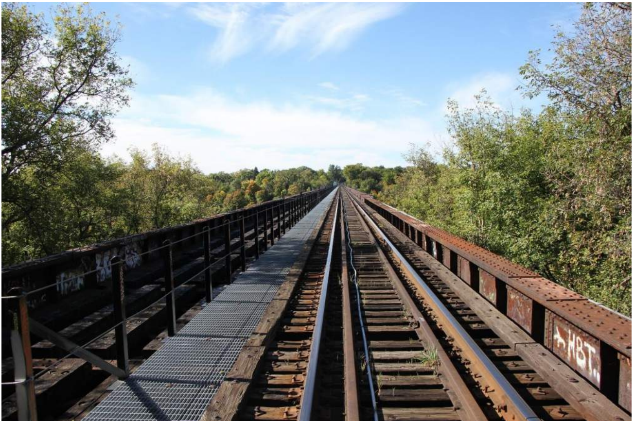
Exhibit B4: Bridge deck looking west
