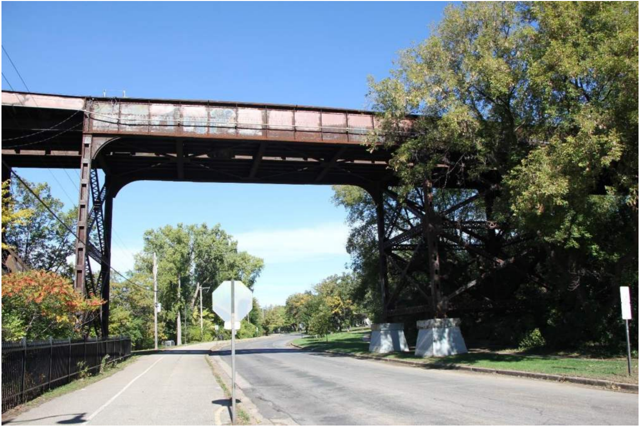
Exhibit B3: Span 5 over East River Parkway looking North
