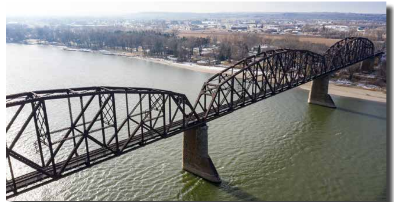
[figure 1.1] aerial drone view of high bridge
