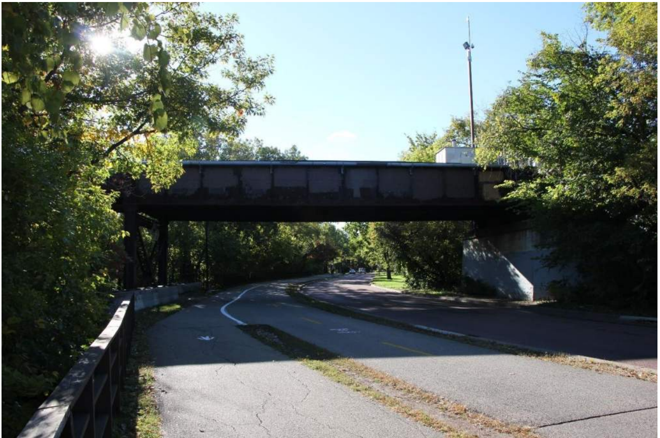
Exhibit B2: Span 1 over West River Parkway looking South
