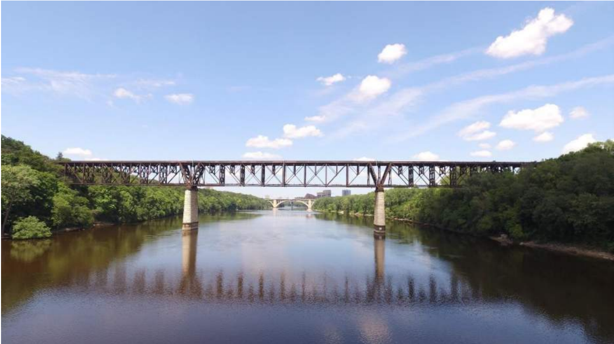
Figure 5: Main Truss Spans 2-4 over River looking North
