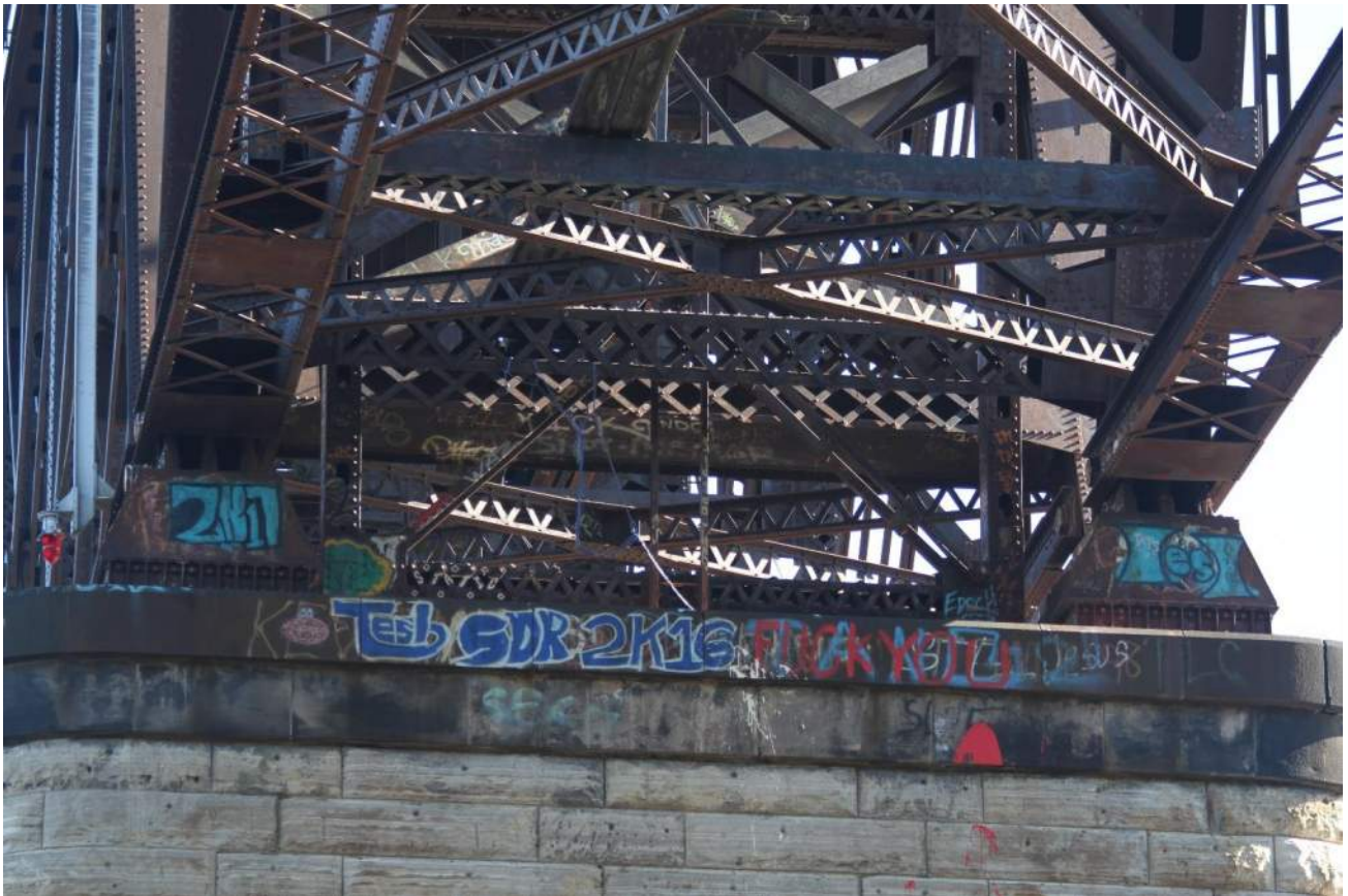
Exhibit B10: Truss bearing at West river pier, looking east:
