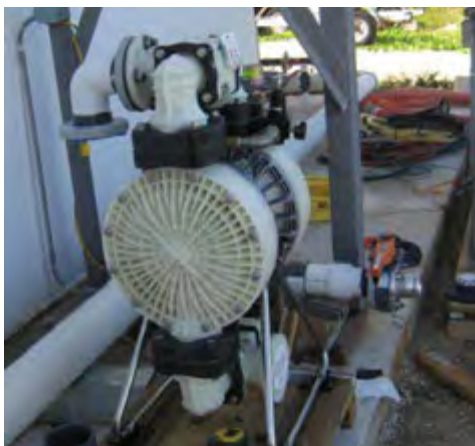
Figure 10. Yamada NDP-80 Air diaphragm pump as installed.
