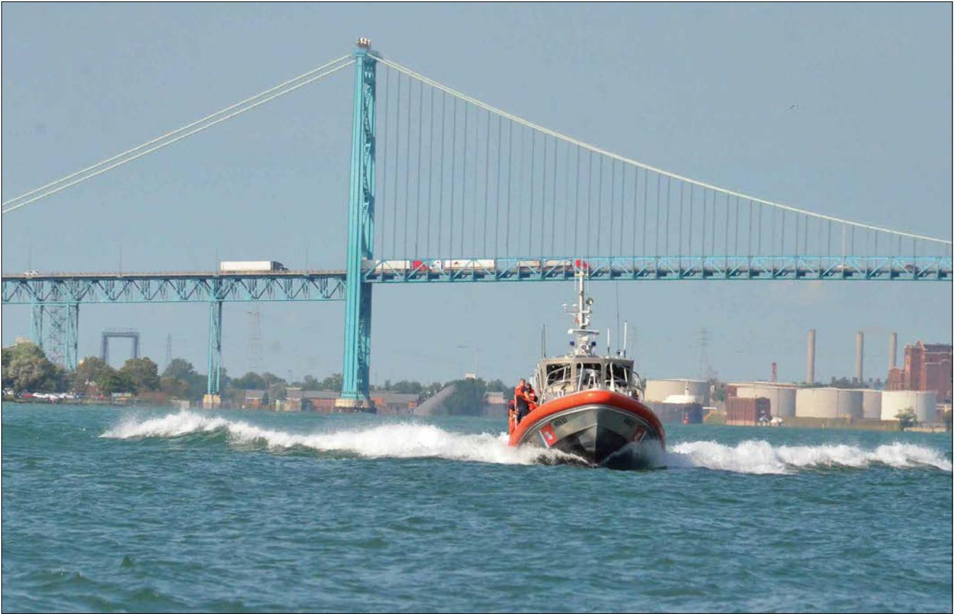
The Ambassador Bridge connects Detroit and Windsor, Ontario, Canada. Between 8,000 and 10,000 trucks transit the bridge each day. Michigan National Guard photo by Specialist Samantha Hall
