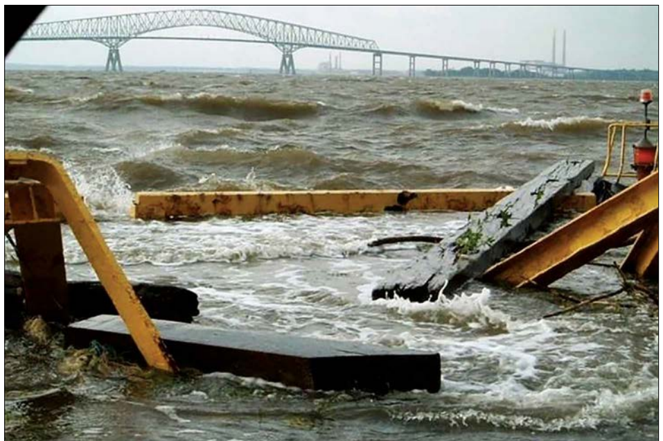
Waves and high water generated by Hurricane Isabel impacted the Port of Baltimore’s Dundalk Marine Terminal in September 2003. The storm produced a surge of 6 to 8 feet at the port and flooded downtown Baltimore. Photo courtesy of the Port of Baltimore
