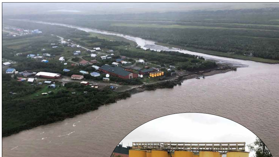
In August 2019, the Lower Kuskokwim School District's fuel storage facility sat just 76 feet from the riverbank's erosion point along Alaska's Kuskokwim River. When the Coast Guard issued an administrative order to the facility's owner, the district, to remove the contents, the tanks held an estimated 36,000 gallons of home heatin oil. Coast Guard photo
