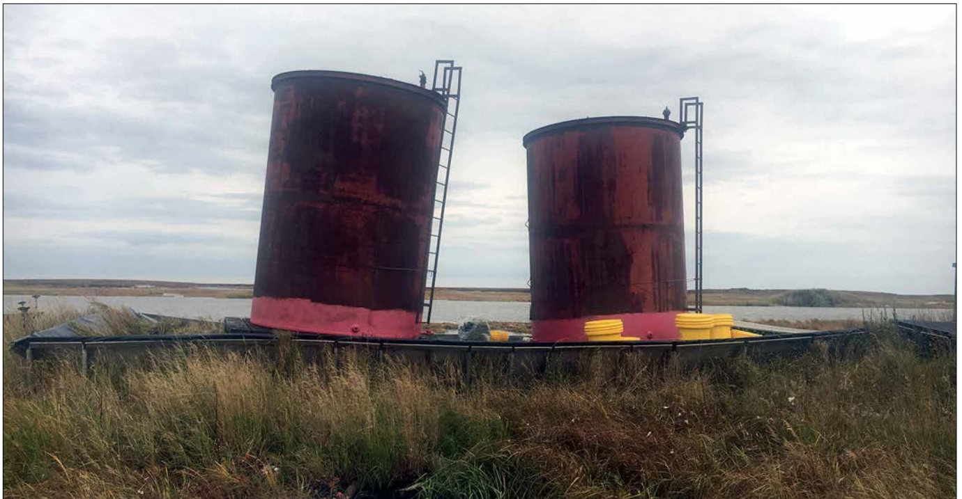
Frost heaves and permafrost thawing threatens fuel tanks like these near Newtok, Alaska, shown in October 2018. Coast Guard photo
