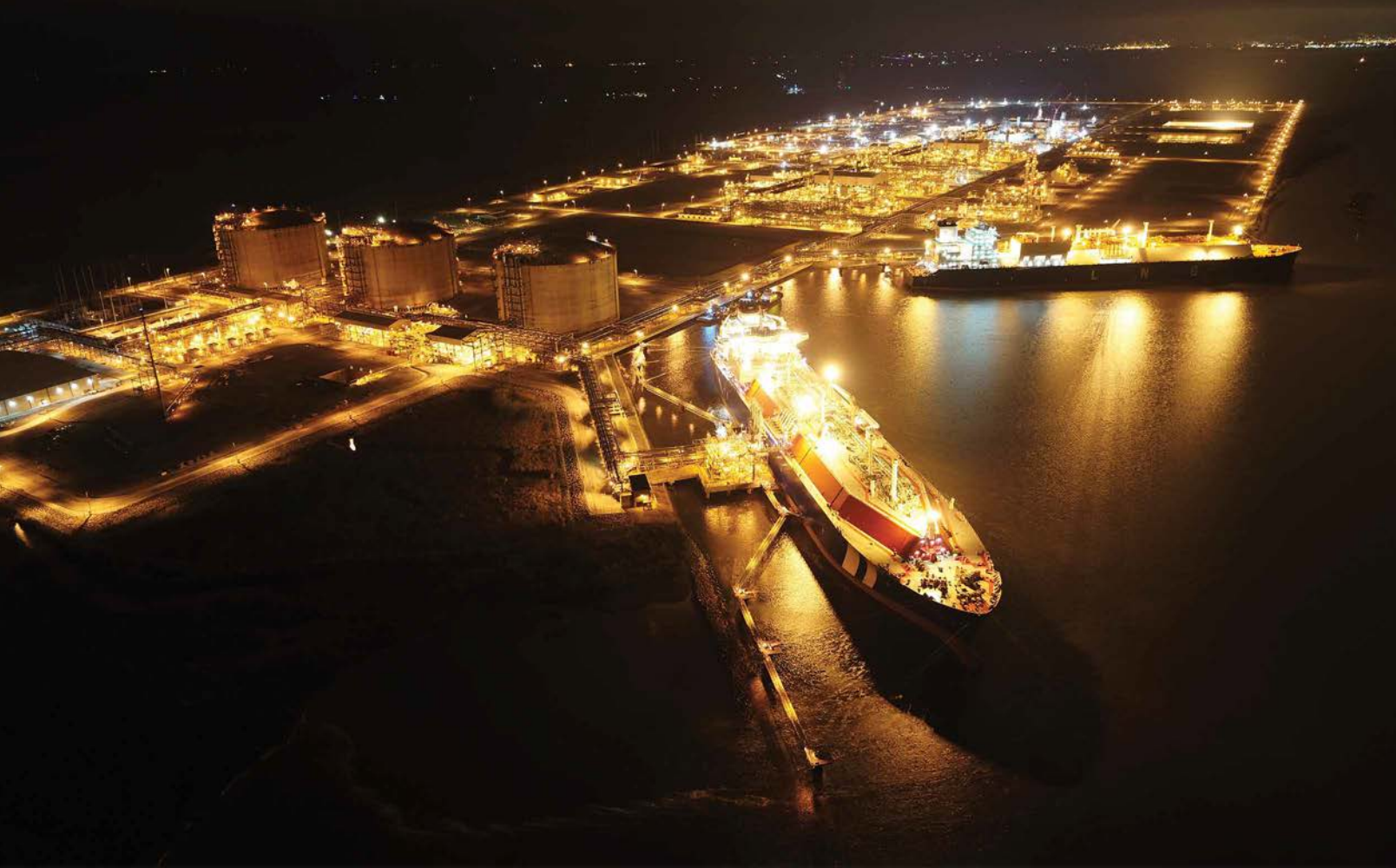
Two ships load liquefied natural gas (LNG) at Cameron LNG's liquefaction facility, where the first two liquefaction trains produce LNG for customers around the world. Photo courtesy of Cameron LNG.
