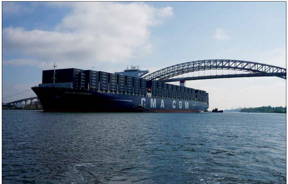
Coast Guard crew members enforce a safety zone in September 2017 as the CMA CGM T. Roosevelt sails under the recently elevated Bayonne Bridge. At the time, the T. Roosevelt was the largest container ship to transit under the Port Authority of New York & New Jersey’s Bayonne Bridge since a four-year navigational clearance project completion. Coast Guard photo by Petty Officer 1st Class Sabrina Clarke
