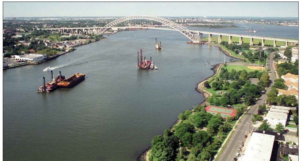
This undated file photo shows three dredges working to deepen the Kill Van Kull, a 3-mile long, 1,000-foot-wide navigational channel that's part of the New York and New Jersey Harbor. U.S. Army Corps of Engineers photo
