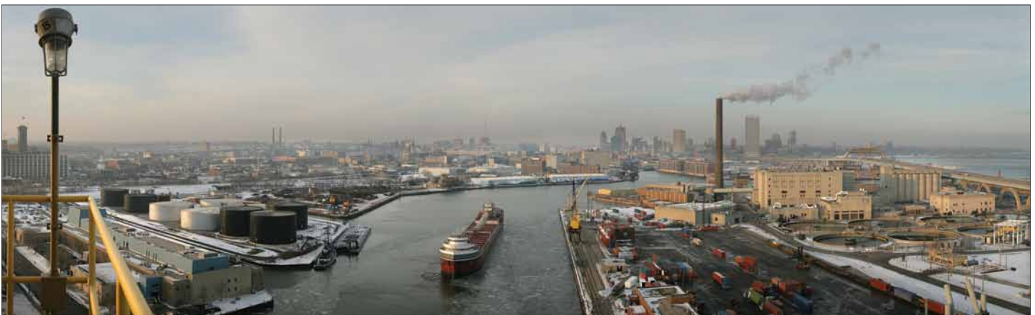
The Port of Milwaukee. Photo courtesy of Discovery World, Milwaukee, Wisconsin.
