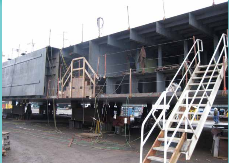
Crowley’s newest double-hulled lightering barge under construction at the shipyard. Photo courtesy of Crowley by Captain Greg Pavellas.
