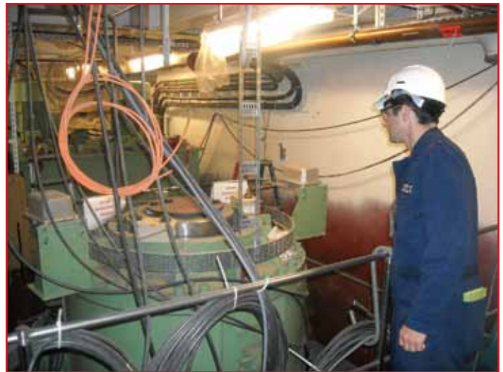
Author LT James Schock, marine inspector, inspects steering gear installation.
