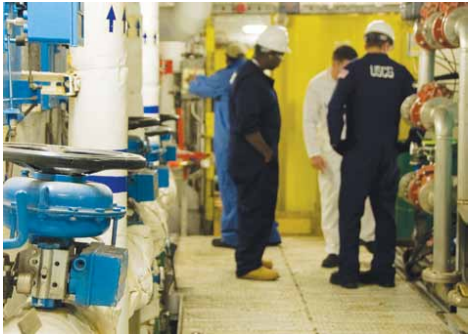
Coast Guard marine inspectors and one of the ship's engineers scan the engine room. U.S. Coast Guard photo by Petty Officer Erik Swanson.
