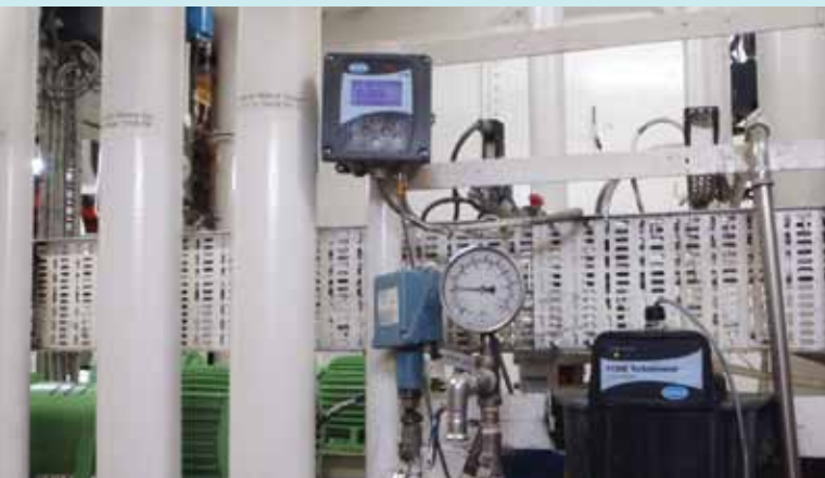
High turbidity could be an “alarm sign” that the treatment process is not functioning well, so a turbid meter can be a valuable process indicator.
