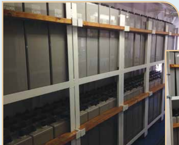
Views of transitional power battery banks.
