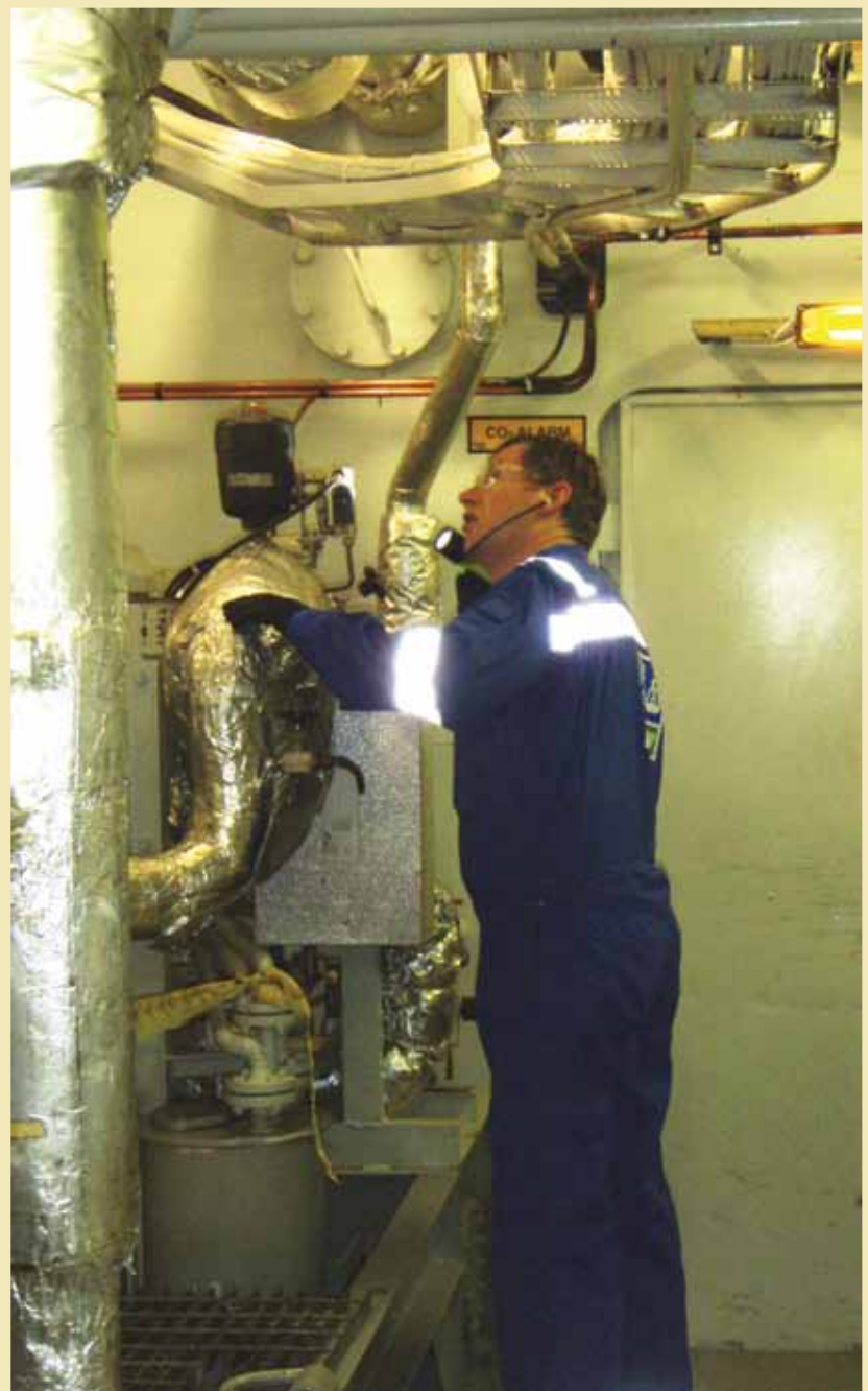
A surveyor witnesses fuel pump remote shutdown.
