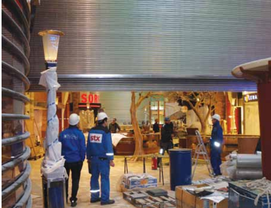
The roller shutter fire door on this cruise ship was the subject of a Regulation 17 analysis. U.S. Coast Guard photo by Mr. Tom Woodford, Marine Safety Center.
