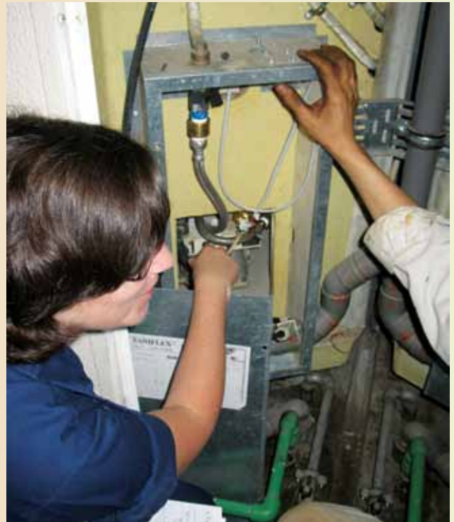
CDR Aimee Treffiletti discusses potable water plumbing with a ship engineer.
