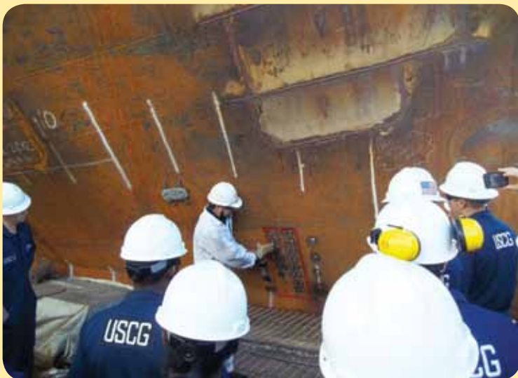
Mr. Marc Cruder, traveling inspector, trains a group of Coast Guard marine inspectors on hull repairs to a sailing barque built in the late 1800s. U.S. Coast Guard photo by MSU Texas City.
