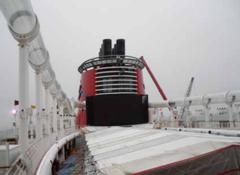
This onboard waterslide passes through structural boundaries. U.S. Coast Guard photo by LCDR Brent Yezefski, Marine Safety Center.
