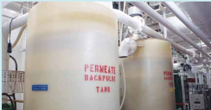
The back pulse system provides suction, moving the water through the membrane.
