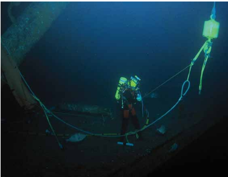
A diver works off of a platform in the Gulf of Mexico. Photos courtesy of Oceaneering International Inc. unless noted otherwise.
