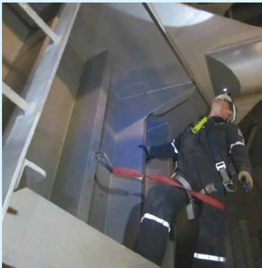
MSSE3 Harley Bates of Sector New Orleans examines internal structural members during an in service inspection program exam.
