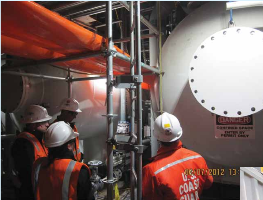
Members of Coast Guard CG-ENG and Sector Puget Sound examine pressure vessel placement aboard a MODU. U.S. Coast Guard photos by Mr. Jay Jerome, Sector Anchorage, Alaska.
