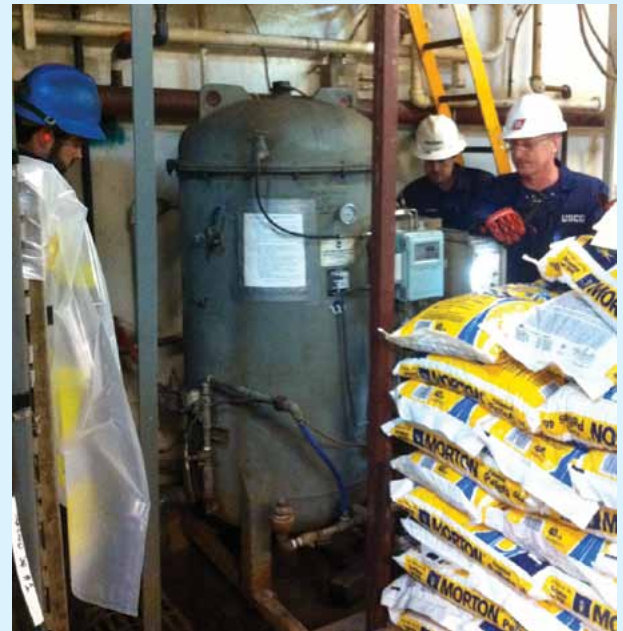
MSSE4 Tony Pesek of Marine Safety Unit Texas City watches oily water separator operation aboard a jack-up MODU.
