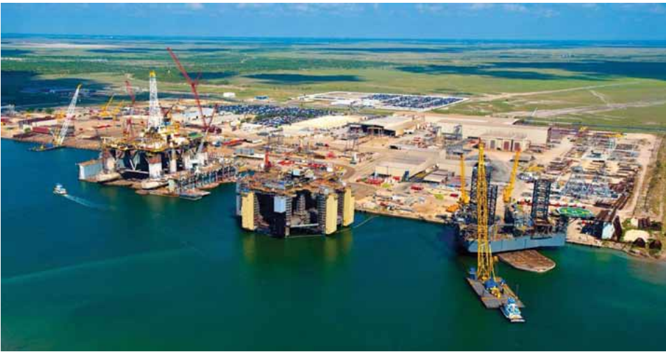
Two semi-submersible MODUs, with one in dry-dock, and a jack-up rig at the KeppelAmFELS facility in Brownsville, Texas. Photo courtesy of the Port of Brownsville.
