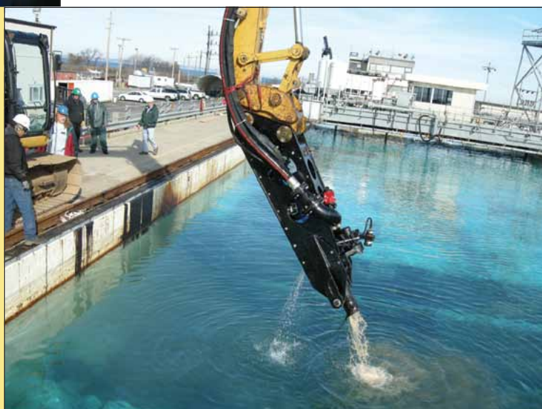
View of excavator-mounted recovery system. U.S. Coast Guard RDC photo.
