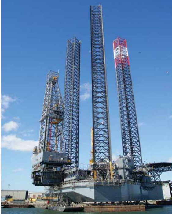
View of drill floor/cantilever on a jack-up rig in Brownsville, Texas. Photo courtesy of the Port of Brownsville.
