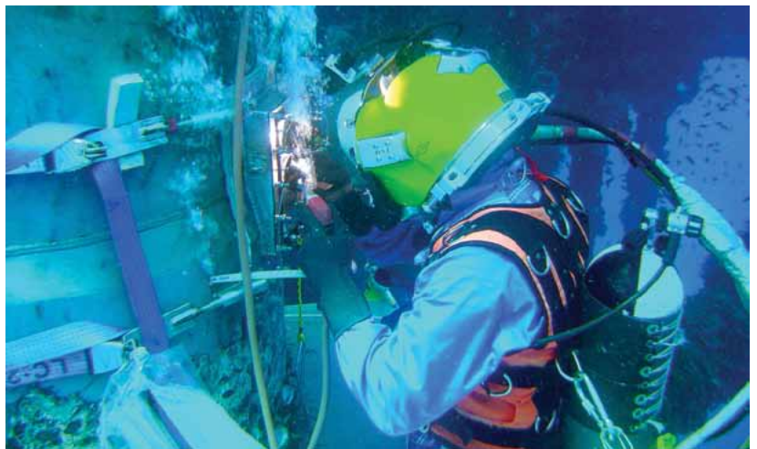
A diver welds underwater on a platform in the Gulf of Mexico. Photo courtesy of Neptune Marine Services.
