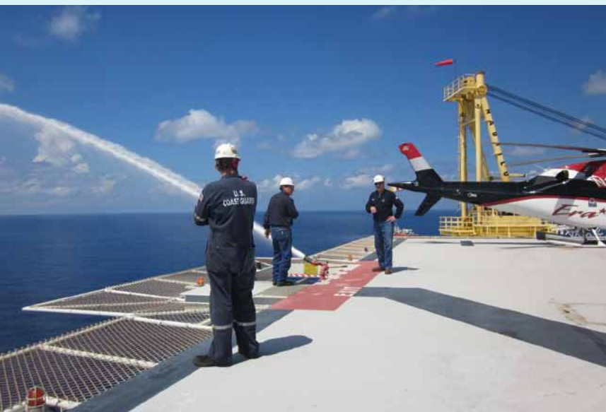
MSSE3 Harley Bates of Sector New Orleans witnesses helo deck foam monitor operation.
