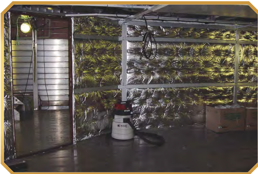
7 KLV SKRWR LQXMDMMV IP SURSHU LQMDMRQRI VVKFWLDO UH SURMFVRQ LQXMDMRQ is excessively compressed in way of pins.
