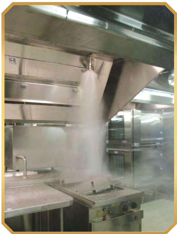
Galley water mist system test.
