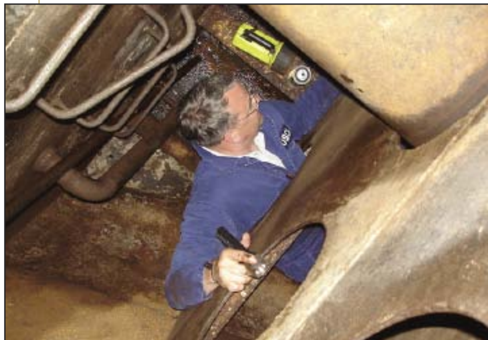
The internal structure, including the tanks and void spaces of an Alternate Compliance and Safety Agreement vessel, is examined by a USCG examiner. USCG photo by Mr. Mike Rudolph.
