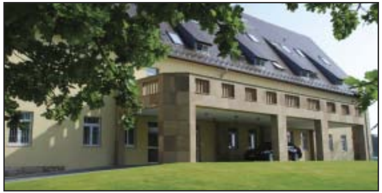
The headquarters of U.S. Africa Command on Kelley Barracks. Kelley Barracks, on the outskirts of Stuttgart, was originally built for the German military in the late 1930s. Photo courtesy of Vince Crawley, U.S. Africa Command.
