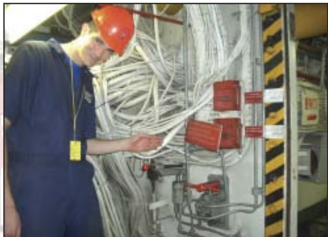
LT Ken McCain of FEACT's prevention department often flies thousands of miles to inspect vessels in other countries. USCG photo.
