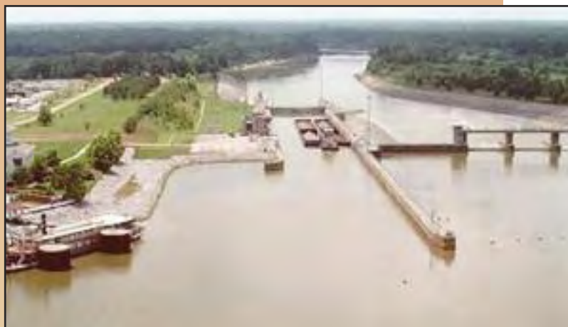
Aerial view of the approach to a lock. In high water conditions, an outdraft current can develop that tends to push vessels off-course toward the dam (right).
