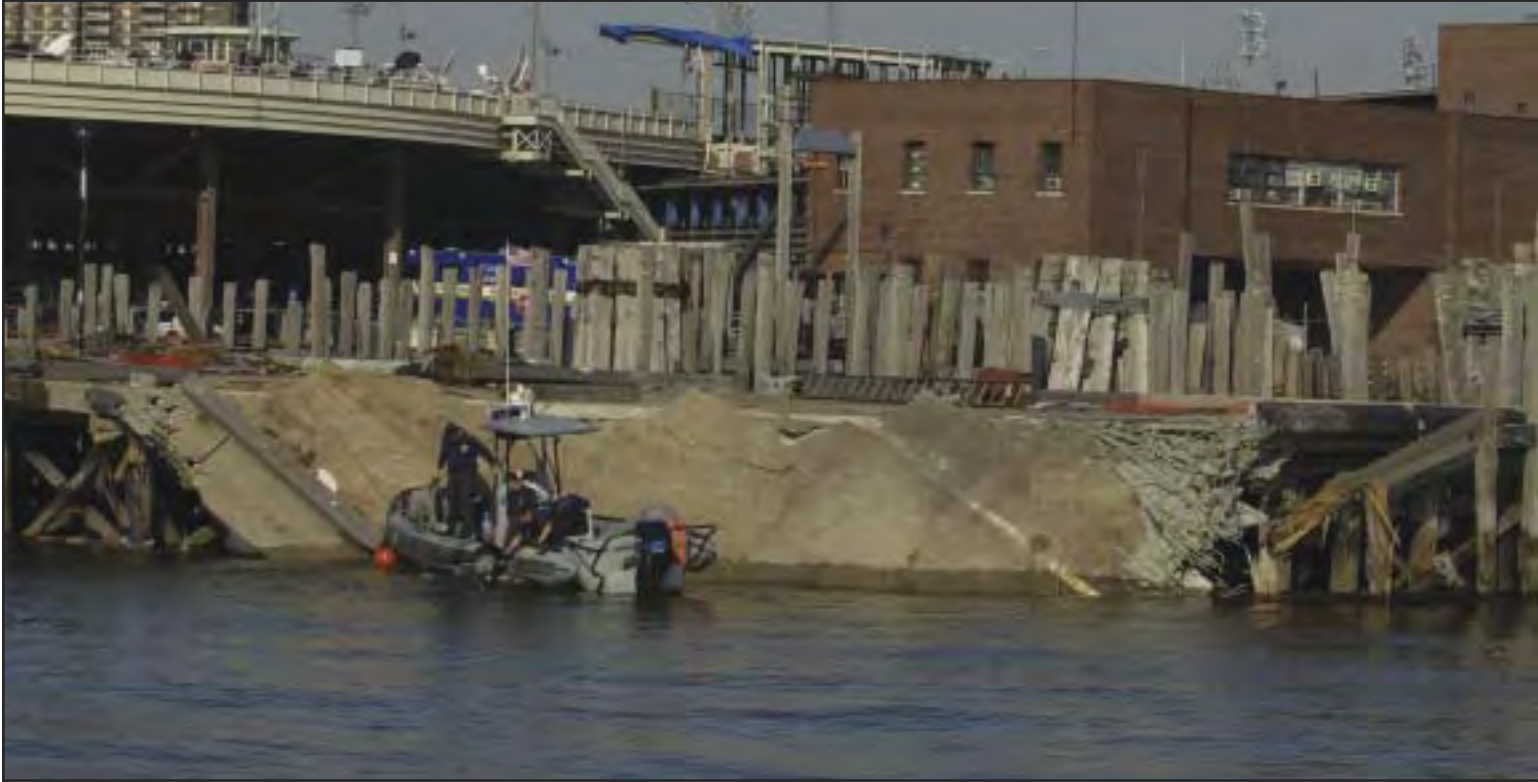
Approximately 1,500 square feet of the maintenance pier surface collapsed into the harbor. USCG photo.
