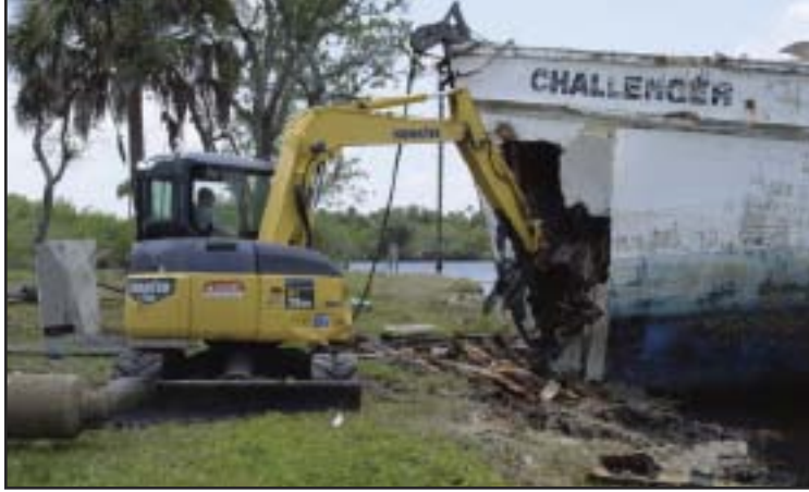
The F/V Challenger's internal structure is demolished and carried away by a backhoe. The primary goal of this process was to significantly lessen the vessel's weight to facilitate lifting by the barge and crane onto shore.
