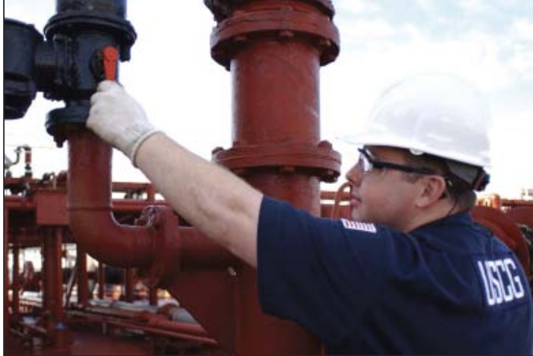
LT Michael Adams, a marine safety inspector from Marine Safety Office Mobile, Ala., inspects for the proper operation of a pressure vacuum valve onboard the 808-foot, Liberian-flagged oil tanker Crude Ocean during a foreign tank vessel exam.
