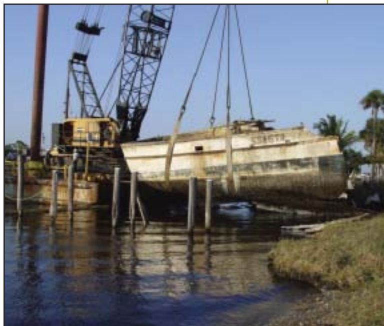
The F/V Challenger's hull is lifted out of the water by barge and crane. All photos courtesy of USCG, taken by MSTC Rafael Tirona.
