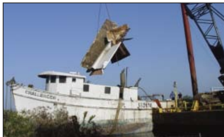
The F/V Challenger 's structure is slowly demolished by barge and crane.
