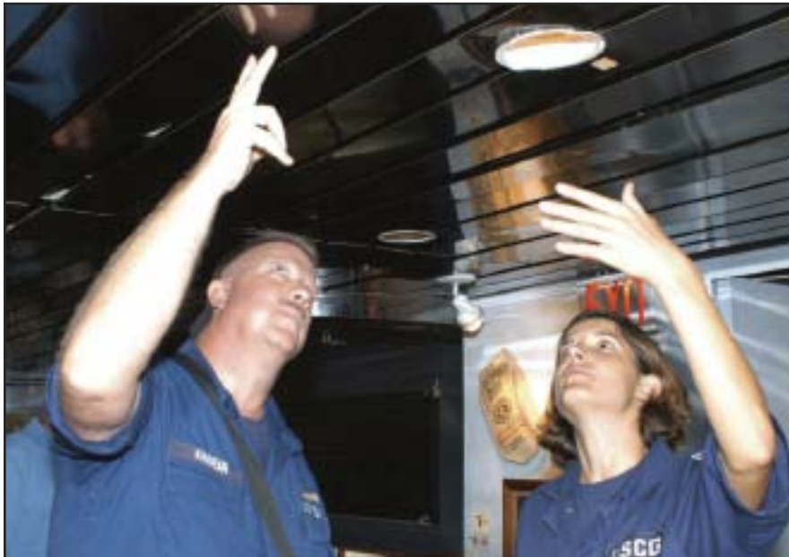
CWO Charles Kinnear, left, from Sector Miami describes the structural fire protection underlying the overhead panel to new inspector LT Josephine Heron during a control verification examination.
