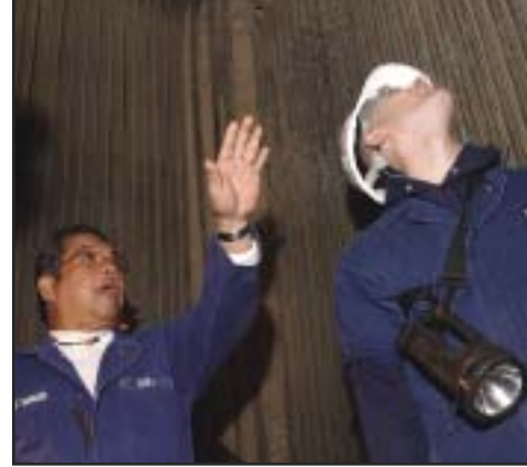
Mr. Cris Cueto, left, instructs LT John Miller on inspecting the inside of a propulsion boiler aboard a steam-powered passenger vessel in New York. USCG photo by PA3 Mike Hvozda.
