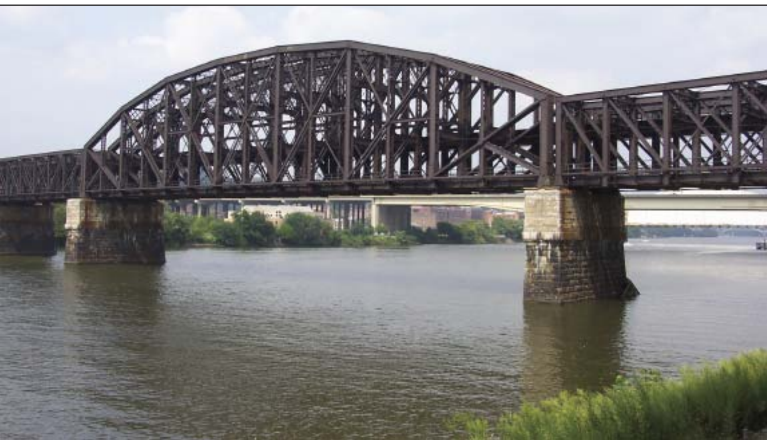
Eleventh Street Bridge, mile 1.0, Allegheny River. USCG photo by W.F. Knutson.
