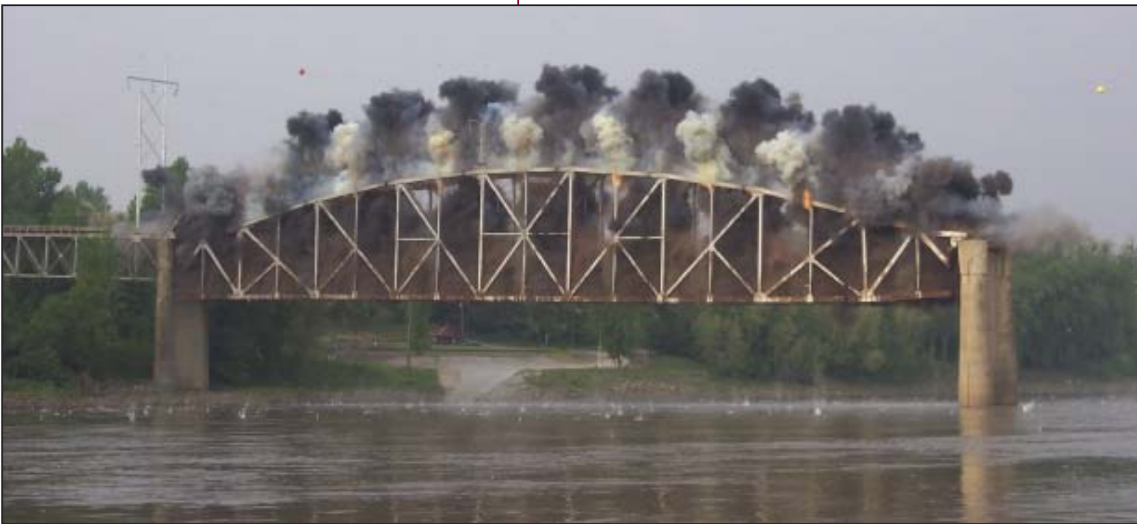
Waverly Bridge demolition, mile 293.4, Missouri River. USCG photo by D.A. Orzechowski.
