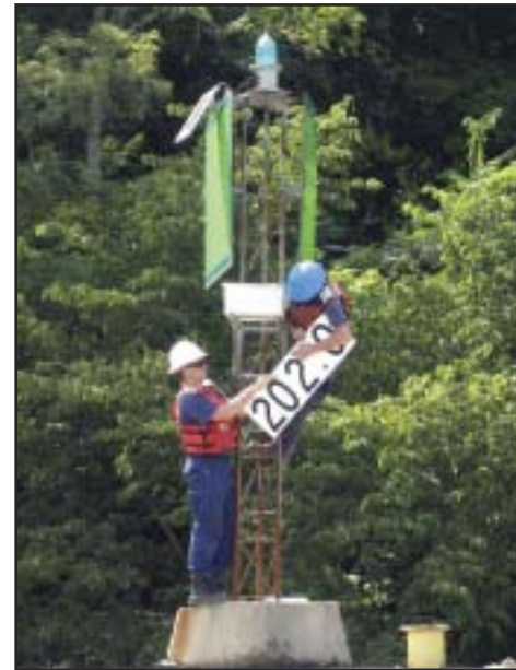
MK1 Benji Mills and SN Trey Cope of USCGC Osage replace the mile board at Blake Run Light on the Ohio River. USCG photo by CDR Kevin Kiefer.
