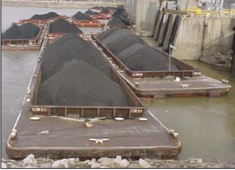
The Racine Lock and Dam allision. Luckily, the barges and dam only suffered minor damage and none of the barges sank or went over the dam. The river was only closed for one day. USCG photo by MST2 Andrew Caldwell.
