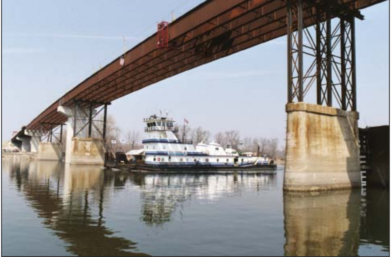
LaSalle Highway Bridge, mile 224.7, Illinois Waterway. USCG photo by W.F. Knutson.
