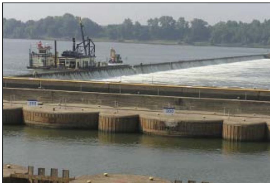
Figure 2: Locks and dam, with the wicket dam raised.
