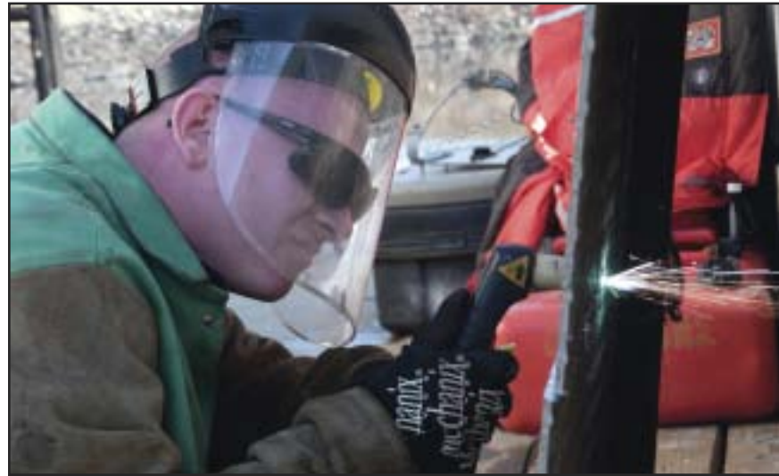
DC2 Patrick Moran conducts maintenance aboard the USCGC Kanawha. USCG photo.
