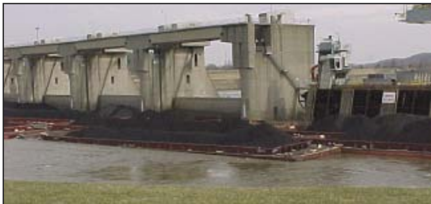
The Racine Lock and Dam located near Letart, W. Va., on the Ohio River. In March 2007, during a period of high water, a towboat lost control and released its tow of fifteen coal barges, which allided with the dam wall. USCG photo by MST2 Andrew Caldwell.
