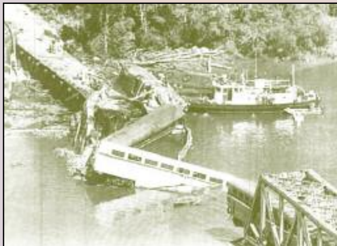
Figure 1: View of the accident site.
