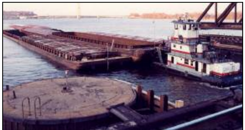
Figure 1: A southbound 15-barge tow transits the Burlington railroad drawbridge, mile 403.1 upper Mississippi River, which provides a horizontal clearance of 153 feet. An assist boat, shown in the foreground, is often used at this bridge. USCG photo by W. F. Knutson.
