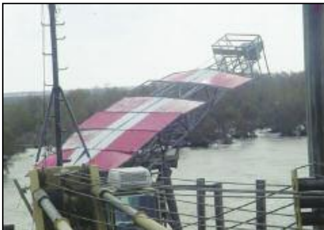
Figure 2: USCGC Pamlico begins repairs to Cubits Gap Rear Range. USCG photo by CWO4 Lewald.
