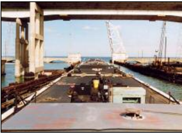
Figure 2: An eastbound tow approaches the Galveston Causeway railroad bridge, mile 357.2 Gulf Intracoastal Waterway. A narrow bridge opening of less than 108 feet, located in an open bay area, results in significant delays due to wind and tide conditions. The highway bridge in the foreground will be replaced with a bridge that will provide about 300 feet of horizontal clearance. USCG photo by W. F. Knutson.
