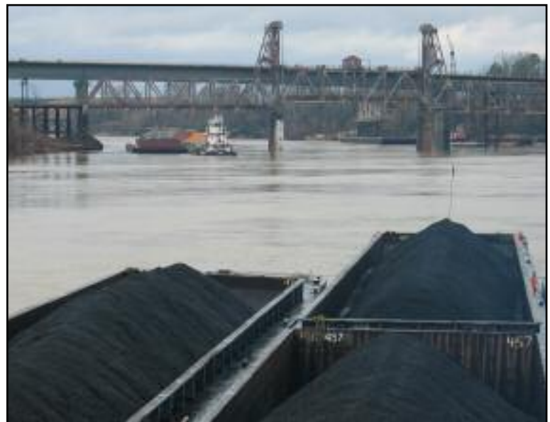
Figure 3: A tow transits a fixed span on the Naheola railroad bridge, mile 173.5 Black Warrior Tombigbee Waterway. Mariners often “double-trip” this bridge during periods of high water. USCG photo by W. F. Knutson.
