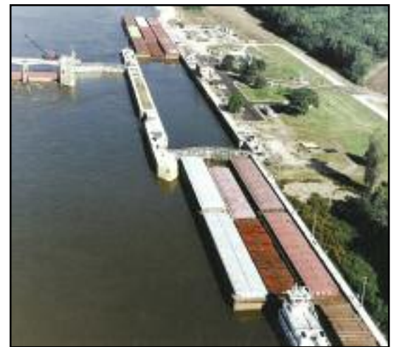
Figure 3: “Double-cut” lockage on the upper Mississippi River. Photo courtesy of the U.S. Army Corps of Engineers, Rock Island District.
