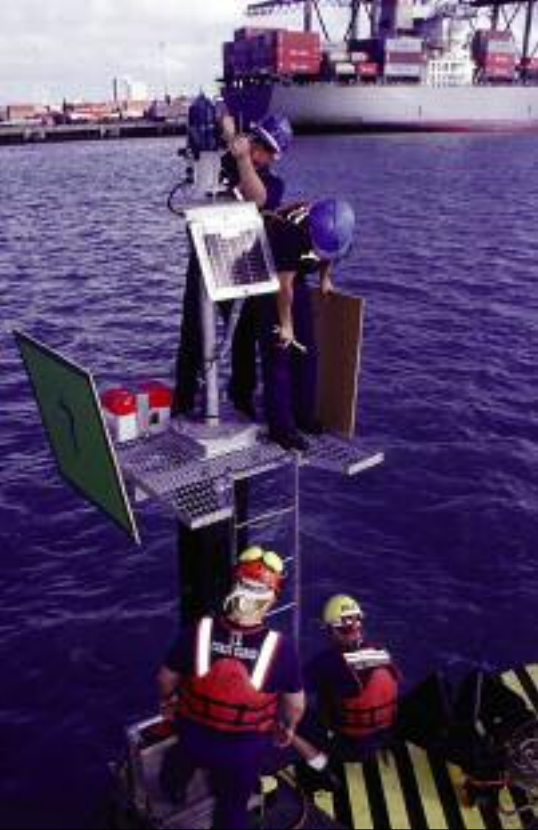
Figure 5: A Coast Guard construction tender putting the finishing touches on a new solar-powered lighted beacon. USCG photo.
