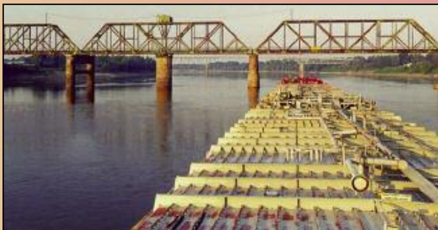
Figure 2: A tow transits a fixed span on the Simmesport railroad drawbridge, mile 4.4 Atchafalaya River. The movable span to the left of the tow is avoided and many mariners opt for a longer route when they cannot transit the fixed span. USCG photo by W. F. Knutson.
