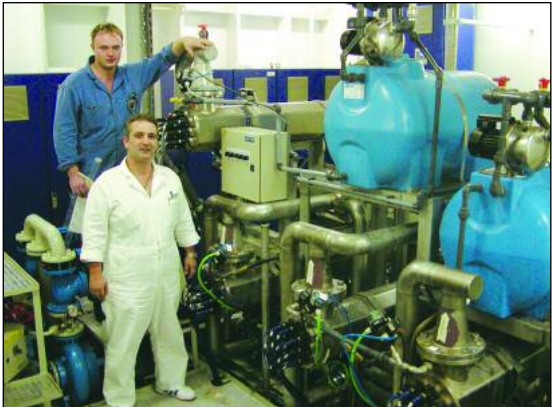
Figure 3: Scanship advanced wastewater treatment system on a Norwegian Cruise Line vessel. Pictured are two shipboard marine engineers charged with running the system. Courtesy Norwegian Cruise Lines.
