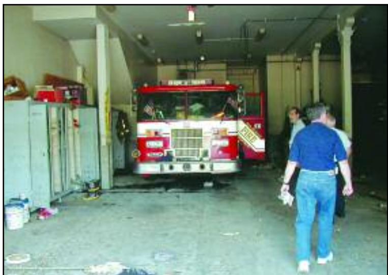
The author documents damage to a New Orleans firehouse where 60-inch floodwaters destroyed two fire trucks and did nearly $500,000 damage to the building.
