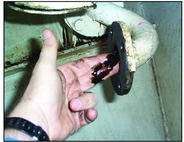
Figure 5: Heavy deposits of oil were found in the pipe leading to the sea.
