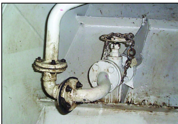
Figure 1: Chipped paint and greasy fingerprints on overboard discharge valve.
