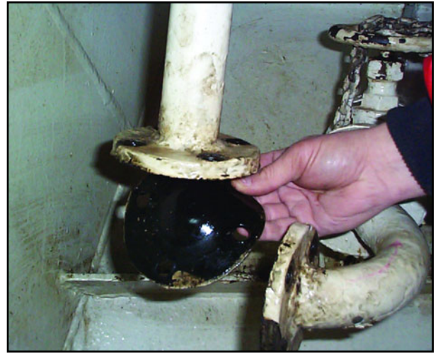
Figure 4: Upon opening piping leading overboard, a blank gasket was found blocking the oil water separator.
