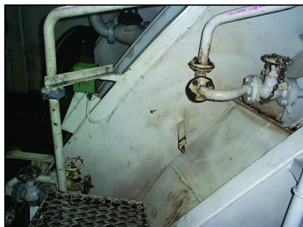
Figure 2: Heavy oil stains on bulkhead and a bracket serving no particular purpose.
