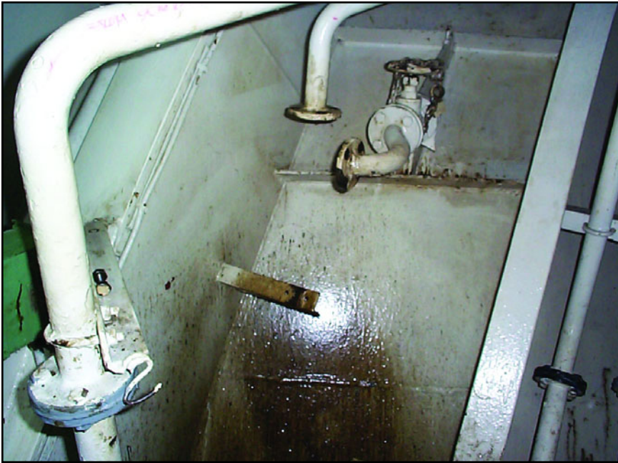
Figure 6: Upon testing the separator, oily water seeped from the separator piping onto the bulkhead.
