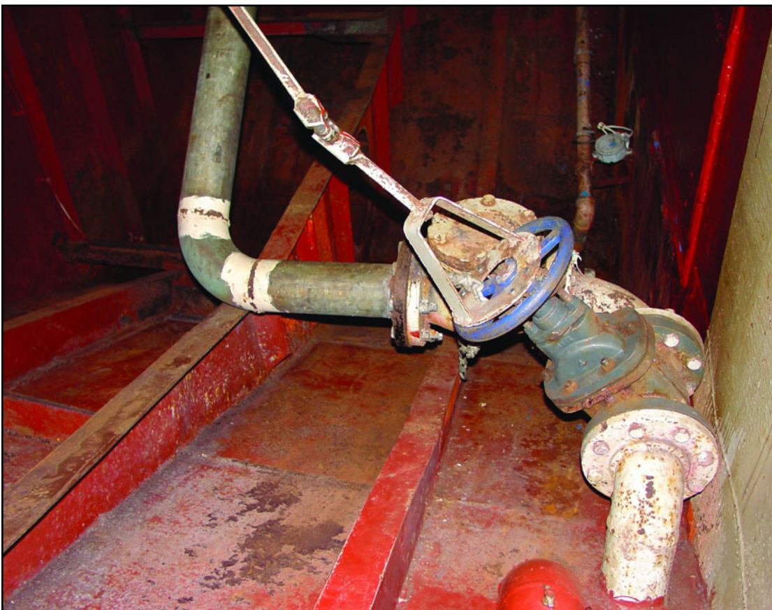
Figure 2: Overboard discharge valve. Dawn M. Kallen, USCG.
