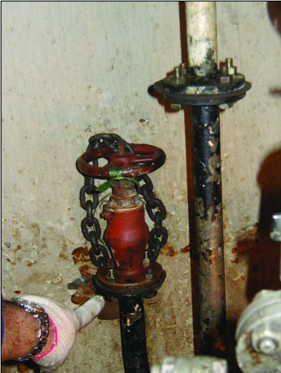
Figure 2: Example of suspicious overboard piping.
