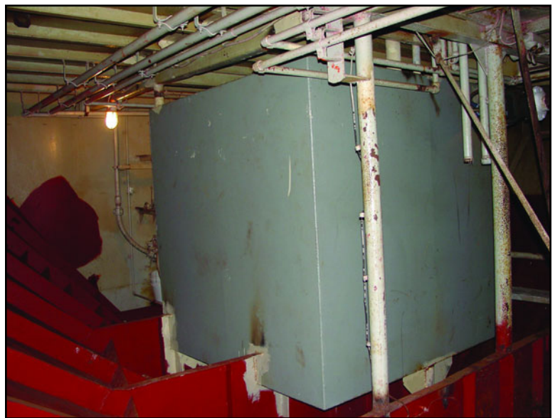
Figure 1: Type III holding tank. Dawn M. Kallen, USCG.
