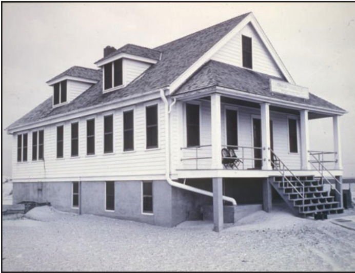
The Pea Island station house.
