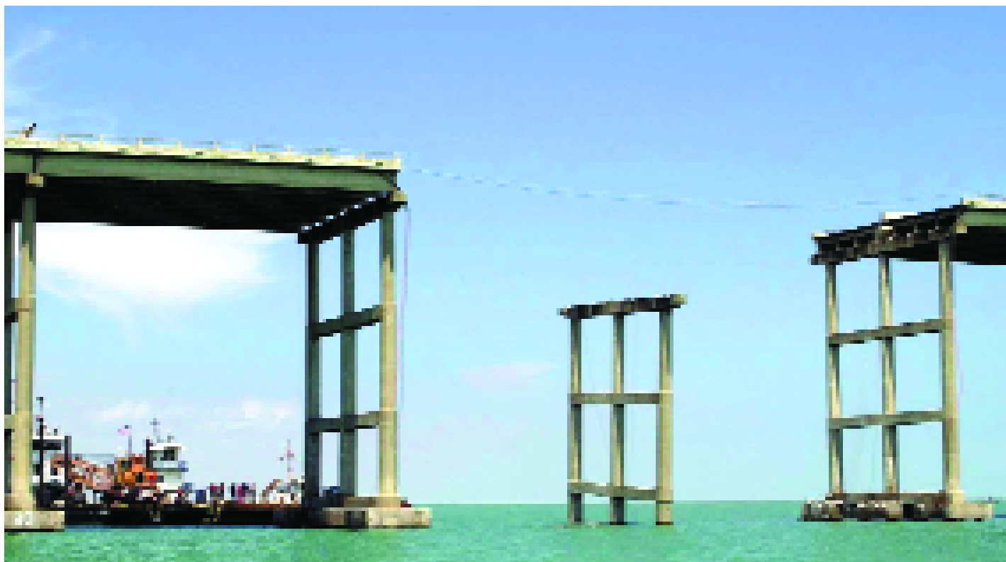
An example of both the human causal factor and group cooperation is the 2001 bridge collapsing in Texas, in which a tug and four barges allided with a causeway, causing 10 cars to fall into the water. Chief Warrant Officer Robert Wyman, USCG.
