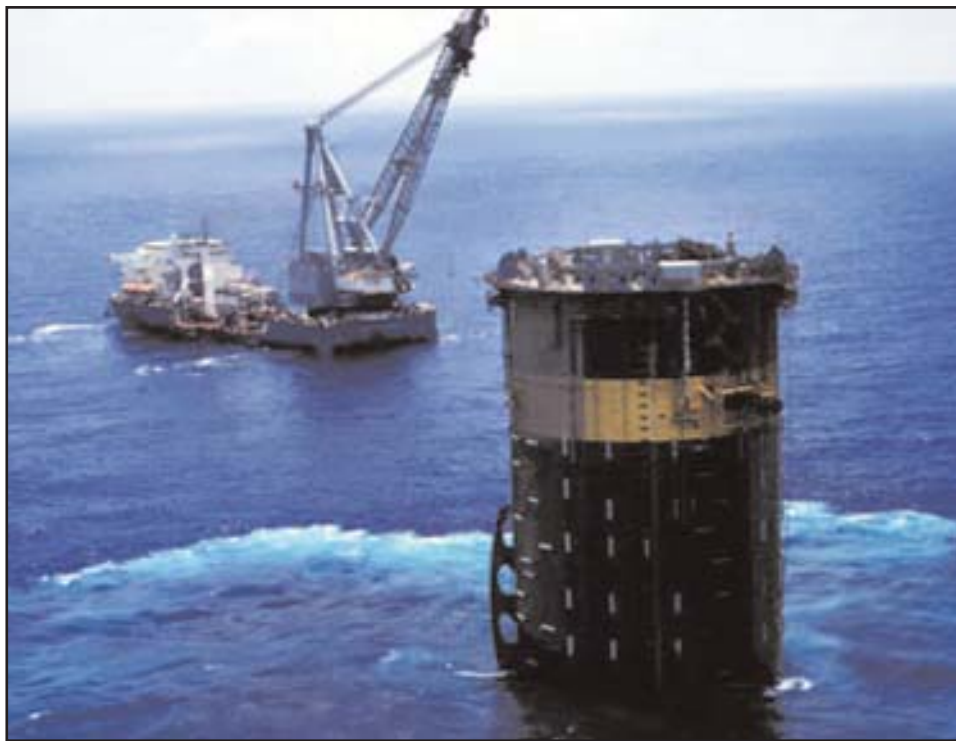
Figure 5. The SPAR’s hull is up-ended once it is in position in its deepwater location. Photo courtesy ChevronTexaco.
