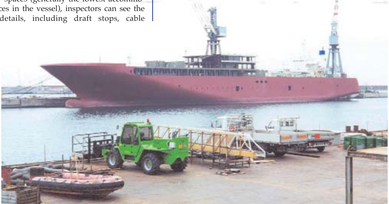
Modular construction of a cruise ship superstructure in Genoa, Italy. USCG photo by Lt. Cmdr. John Mauger.
