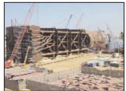
Figure 2. A truss SPAR design. USCG photo by Lt. Bryan Dunlap.
