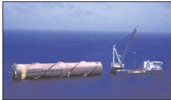
Figure 1. A solid continuous steel hull designed SPAR. Photo courtesy ChevronTexaco.
