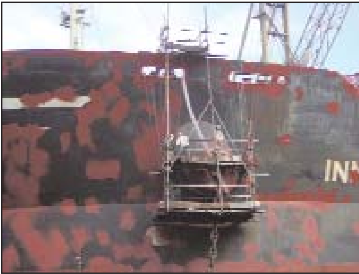
Chain scaffolding attached to the back of a vessel in a Singapore yard for a rudder repair. USCG photo.
