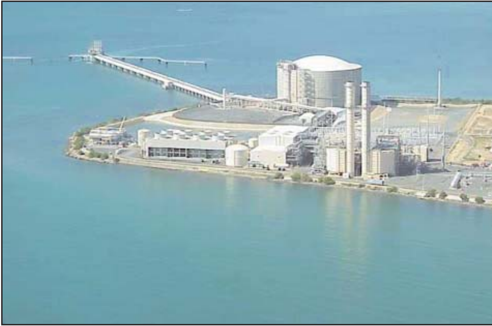
An LNG facility in Guayanilla, Puerto Rico. USCG photo.
