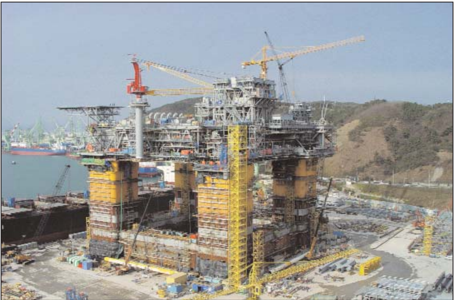
Completion of NaKika, which is in production, is expected in late 2003. The platform is designed to process 425 million cubic feet of gas and 110,000 barrels of oil per day. Photo courtesy Shell Oil Co.
