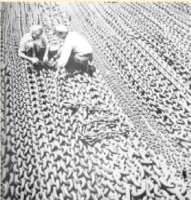
Coast Guardsmen check moorings for buoys and light-ships (Nov. 1944).
