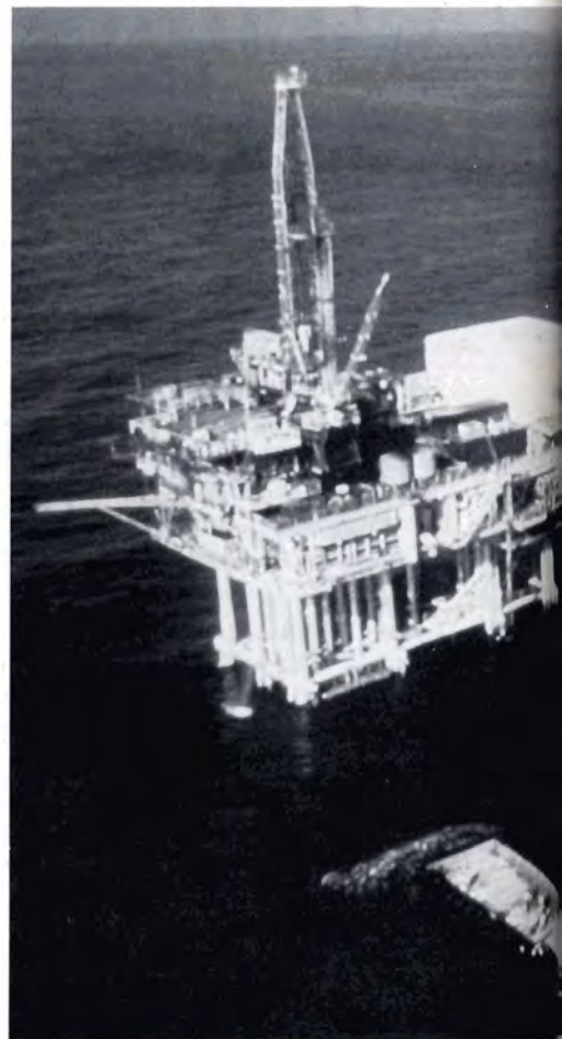
Drilling and production facilities.
