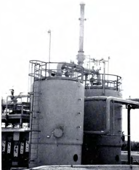
Unit liquefies vapors for easy recovery.
