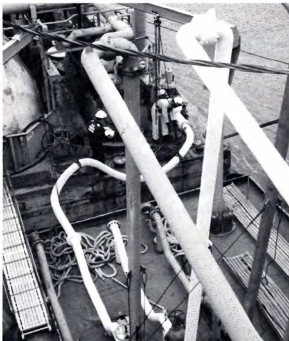
Tanker operator hooks up lines to transfer anhydrous ammonia.
