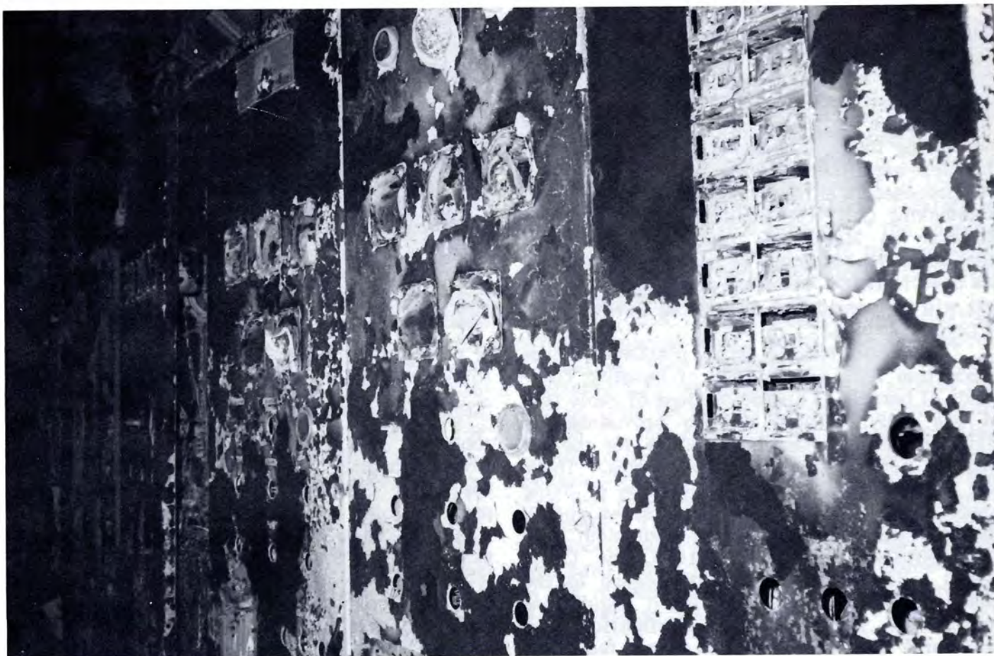
The gauge board inside the generator room bears mute witness to the fire's severity.
