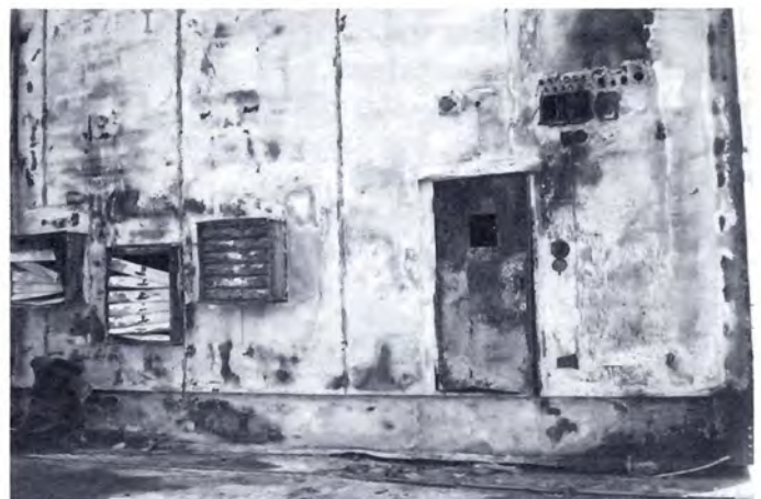
The intensity of the explosion and fire caused this damage to the generator wall facing the living quarters. (All photos are from U.S. Coast Guard files)
