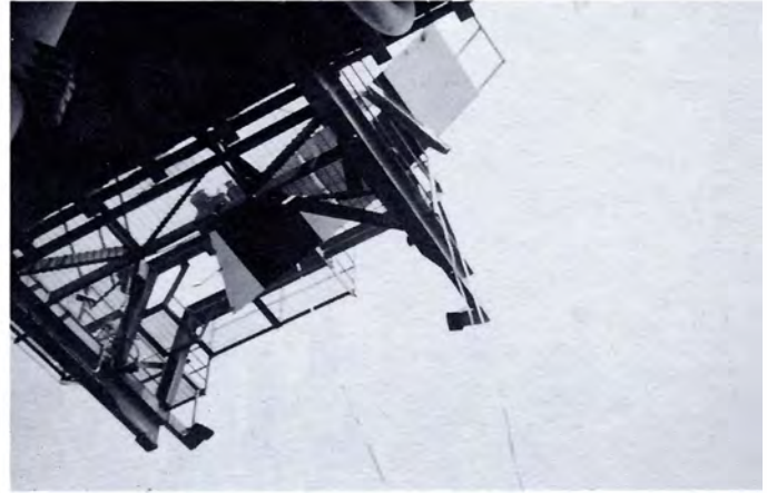
A portion of the helo deck was blown into the life capsule support frame by the explosion.
