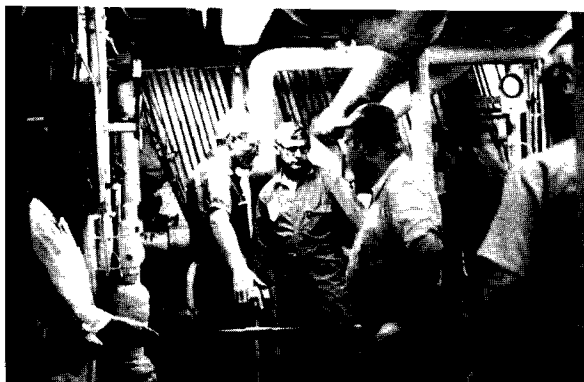
The engine room presents special hazards. Trainees check their knowledge of equipment and techniques.
