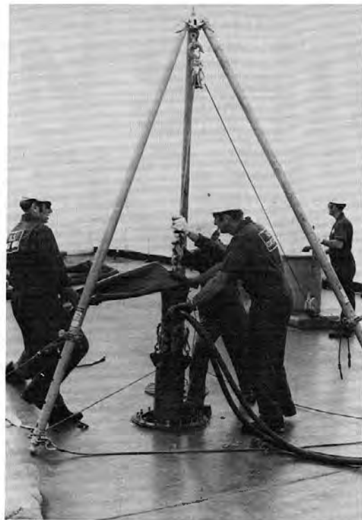
Members of the Coast Guard's National Strike Force prepare to pump cargo from the SHOWA MARU's damaged cargo tanks using their portable, hydraulic driven, submersible transfer pumps. The men and equipment were brought from as far as North Carolina; other pumps were transported from Virginia.
