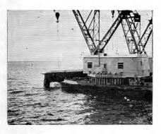
Once all vessels were upwind, the cranes took a strain and began the righting operation. Shortly after the barge began to turn, however, one of the wire cables parted at the point where it passed over the intersection of the bottom and side of the barge. That portion of the wire cable was replaced with chain, and the barge was slowly turned.
