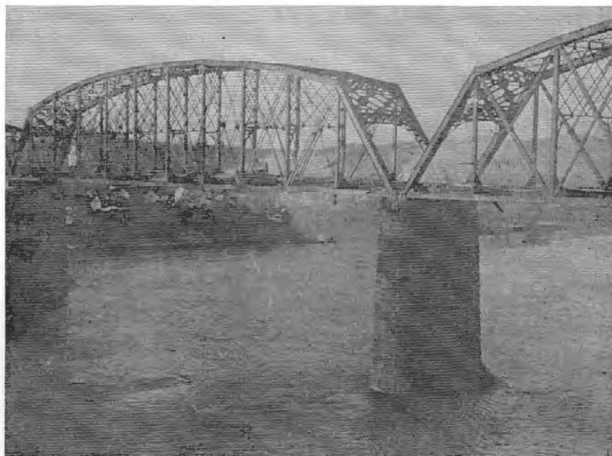
Damage to the bridge at Parkersburg was estimated at $1 million. Replacement rather than repair of the span that suffered the effects of the explosion was deemed the most efficient method of returning the bridge to service.
