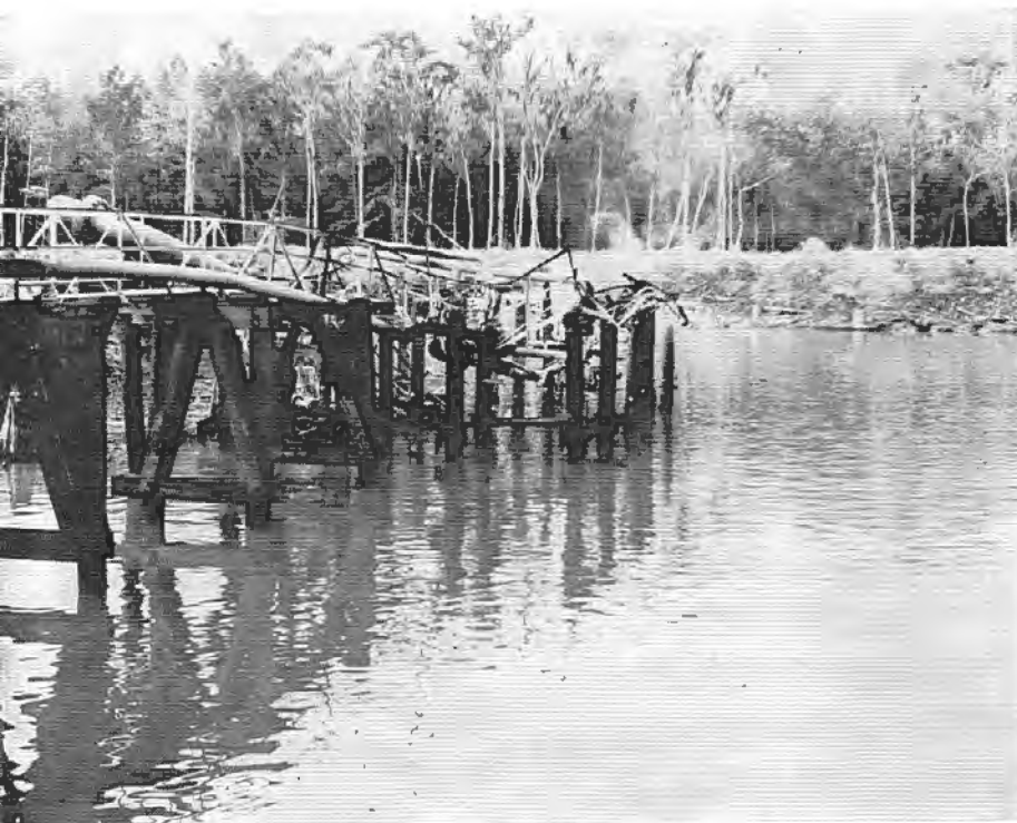
In this picture, taken from the barge, is shown the damage to the railing structure and the pipeline that leads from the shore to the barge loading terminal. Parts of the structure are still smoldering, as manifested by the smoke rising at the center of the picture.
