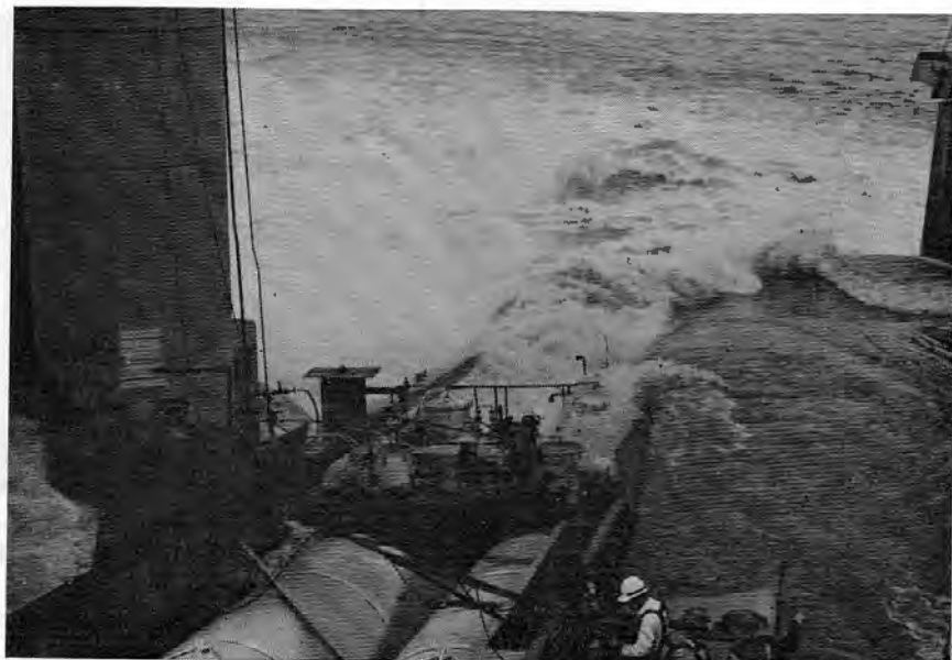
Improvised but effective splash shields protected the hatch cover area of the barge from the torrents of water that raced through the spillway while the offloading operations were underway. The splash shields can be seen on each side of the hatch cover area in this photo.
