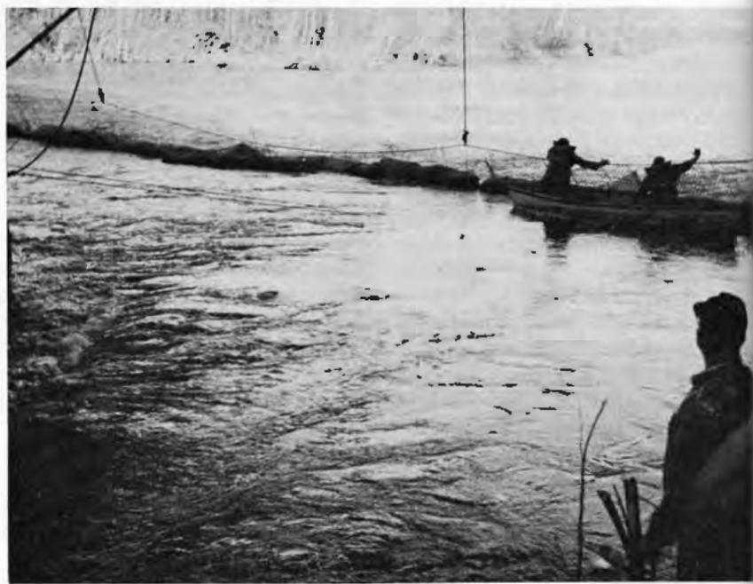
AN OIL SPILL in the Schuylkill River near Philadelphia in November of last year prompted many makeshift attempts at containment. This one involved absorbent materials retained by chicken wire and suspended from a bridge overhead.
