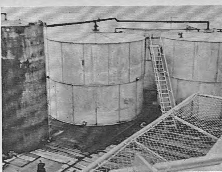
Pictured above is the Chambers and Kennedy Offshore Oil Platform before the casualty. At the far left is the "gunbarrel"; center is Number 1 storage tank; right is number 5 storage tank. A welder struck an arc on the equalizing line above the ladder to the tank tops, setting off the explosions and fire.
