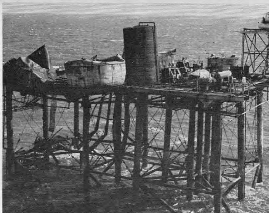
The Chambers and Kennedy platform was extensively damaged by the explosion and fire on 28 May 1970. Damage to the structure was estimated at $200,000.
