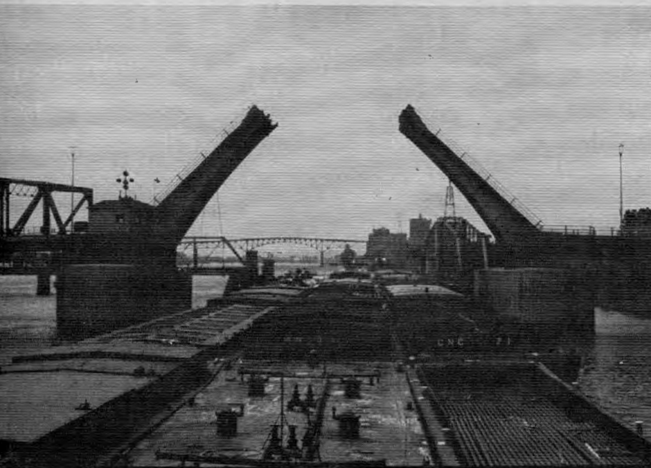
SLOW PASSAGE and caution are necessary here. The opening provided by the double-leaf bascule bridge is narrow, and a railroad swing bridge is close at hand.
