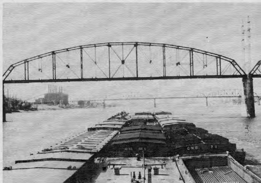
A THROUGH truss railroad bridge spanning the Mississippi at St. Louis. Vertical clearance is 44' at high water.
