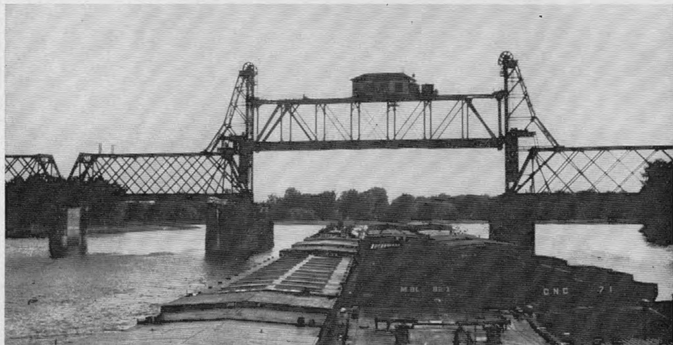
BRIDGES OVER navigable waters must be constructed with the needs of navigation in mind. In this case, a vertical lift railroad bridge over the Illinois River, the raised lift span provides for overhead clearance.
