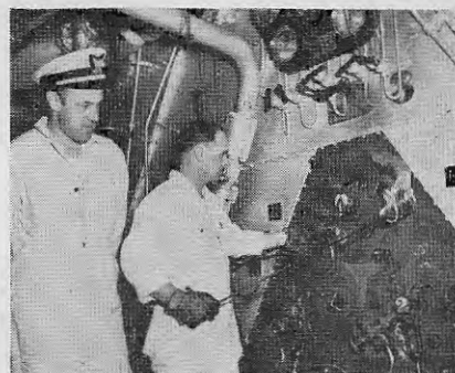
SHIP'S FIREMAN lights off a boiler for the Coast Guard inspector.
