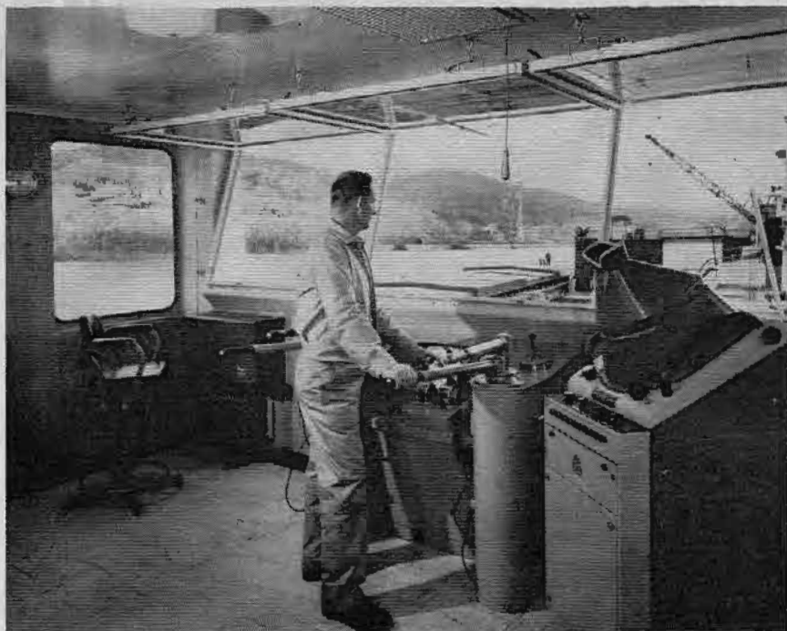
Pilothouse on a modern river towboat is designed for maximum visibility and is equipped with all modern navigational aids including radar and ship-to-shore radiotelephone.
