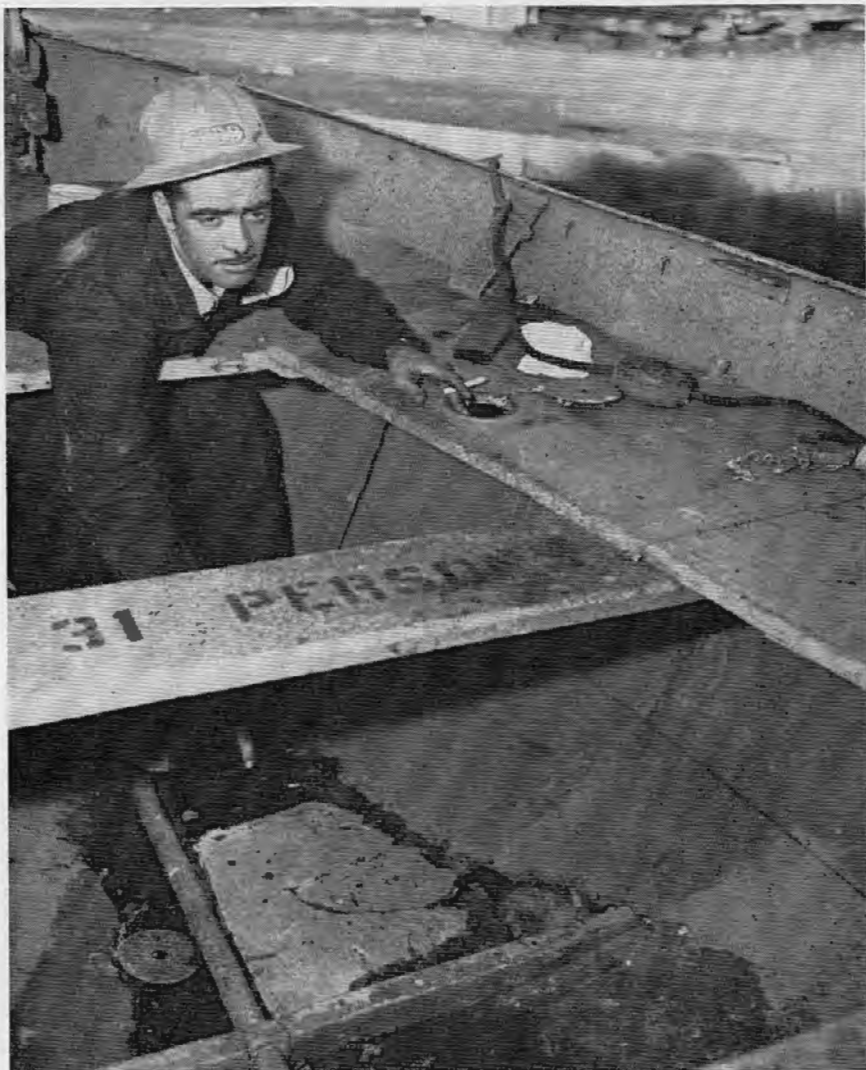
THIS IS MAINTENANCE? A shipyard employee is pointing out a cement patch in the bottom of a lifeboat. This "repair" was discovered at a Coast Guard inspection, although no repair item was considered necessary or included on the worklist.
