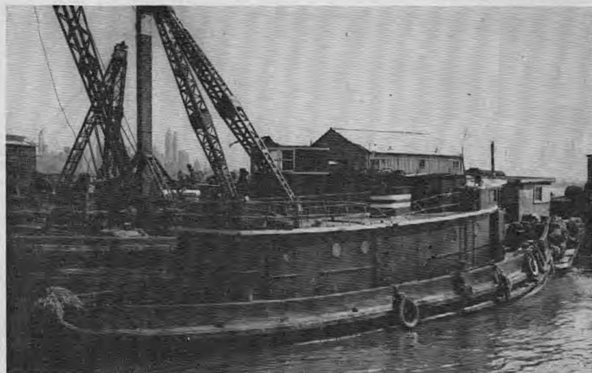
Figure 3. View of tug a short time after it was refloated. Note the low center of gravity—nevertheless she capsized, mainly because she was underpowered.
