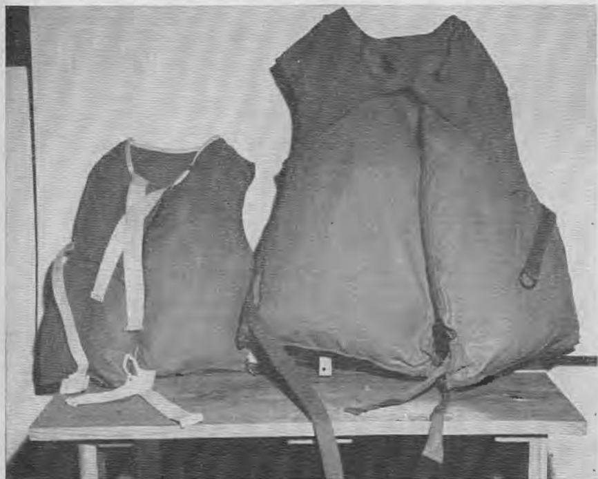
FIGURE 2 illustrates two typical approved jacket-type life preservers. Each approved jacket-type preserver must be stamped ADULT or CHILD, as the case may be, and in addition with the Model No., Manufacturer's Name and Address, Coast Guard approval number, and that it has been PASSED by the inspector.
