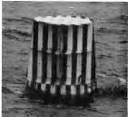
FIGURE 3.—"XRA" Type can buoy.
