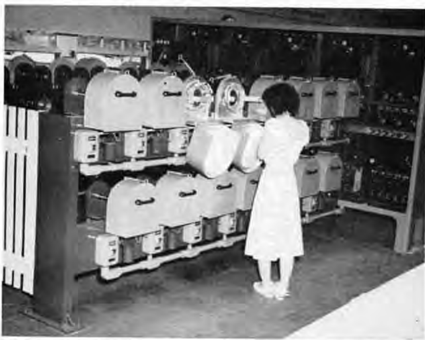
FIGURE 9.—Some of the high-speed spindles for testing greases in roller bearings at various temperatures, U. S. N. Engineering Experiment Station.
