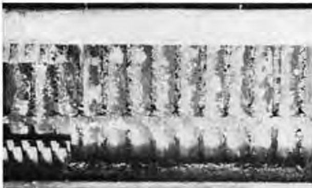
FIGURE 1.—Tube bank before typical water-cleaning operation.
