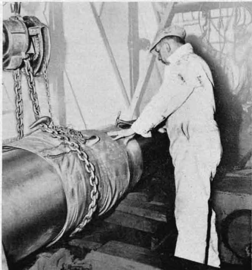
Marine Inspector checking propeller shaft liner.
