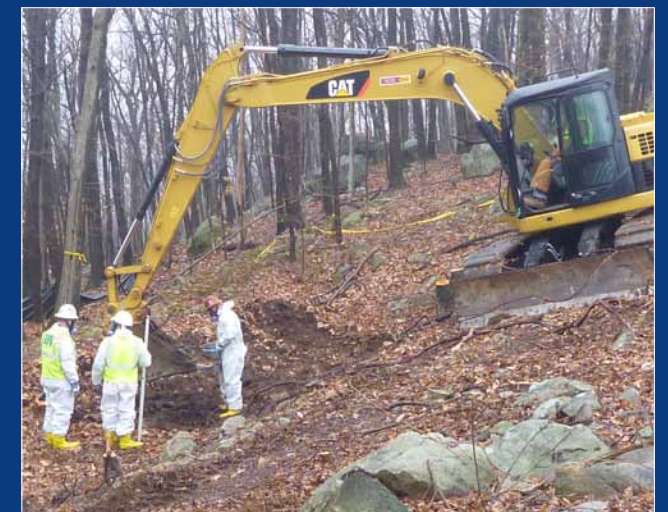
Contractors work to excavate hazardous material that seeped into the soil and groundwater over the years, Feb. 24, 2012. U.S. Coast Guard photo by Petty Officer 2nd Class Jonathan Scott.
