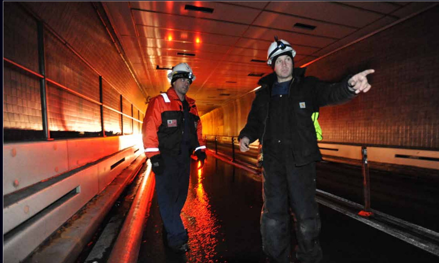
Petty Officer 1st Class Eugene Peters and Petty Officer 2nd Class Austin West conduct dewatering operations inside the Hugh L. Carey Tunnel in New York City, Nov. 9, 2012.
