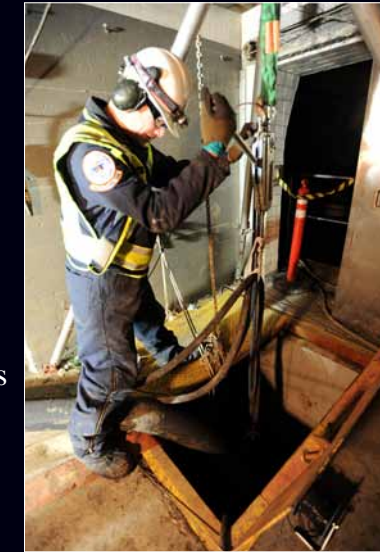
Petty Officer 2nd Class Karl Siegmund works the rigging of a submersible pump inside the tunnel in New York City, Nov. 9, 2012.
