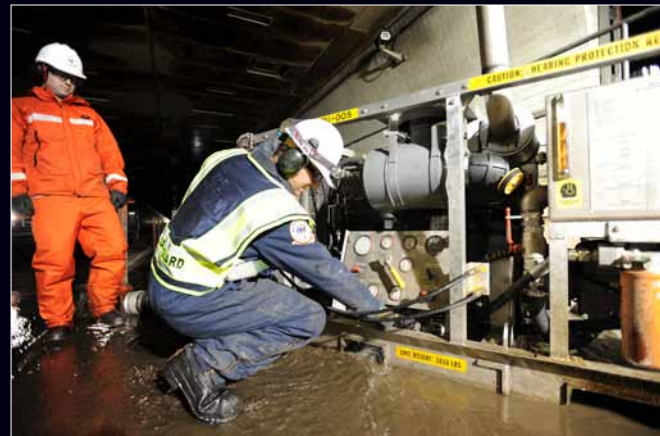
Petty Officer 2nd Class Jeffrey Burby and Petty Officer 2nd Class Karl Siegmund monitor a hydraulic prime mover while conducting dewatering operations at the tunnel in New York City, Nov. 9, 2012.
