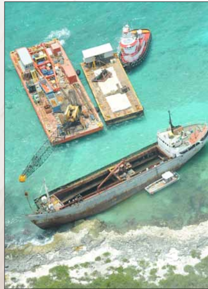
Response crews cut and remove sections of the Jireh for removal and disposal, Aug. 18, 2012. U.S. Coast Guard photo by Petty Officer 2nd Class Jaclyn Young.
