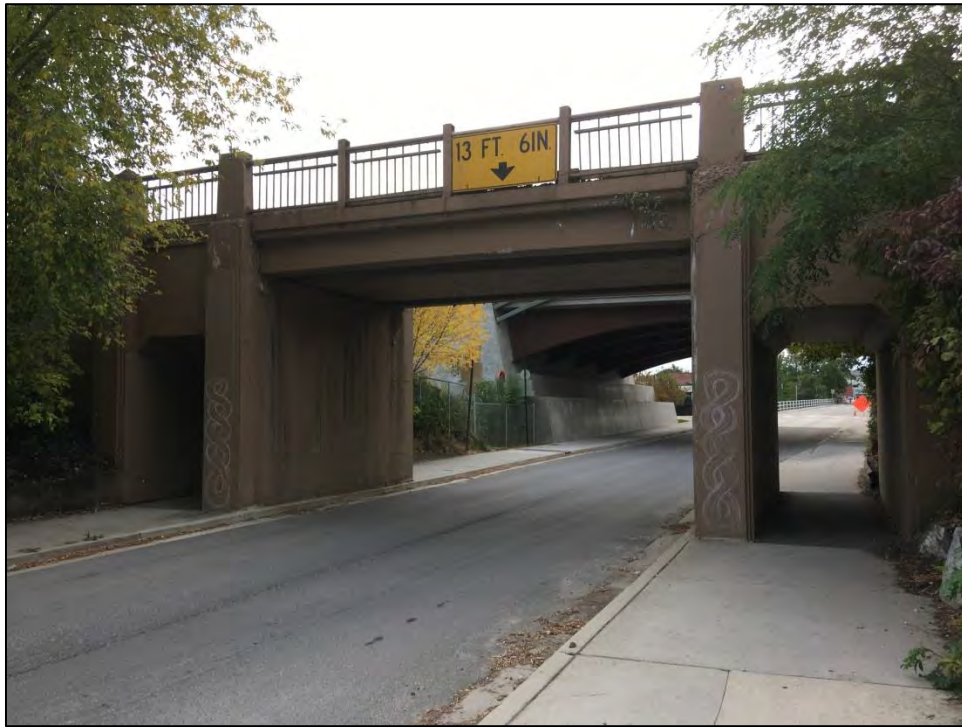
Figure 28. BNSF Bridge 3.0 West Elevation
