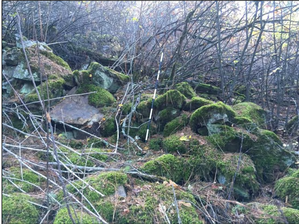
Figure 6. Wall profile near eastern end; view southeast.
